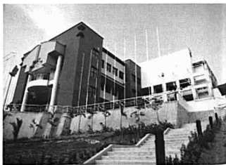
The administrative block at the State Stadium at Petra Jaya.
