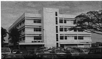
The newly constructed Specialist Clinic at Sarawak General Hospital.
