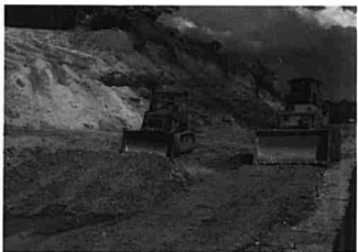
Road Construction - to link up the rural population centres.
