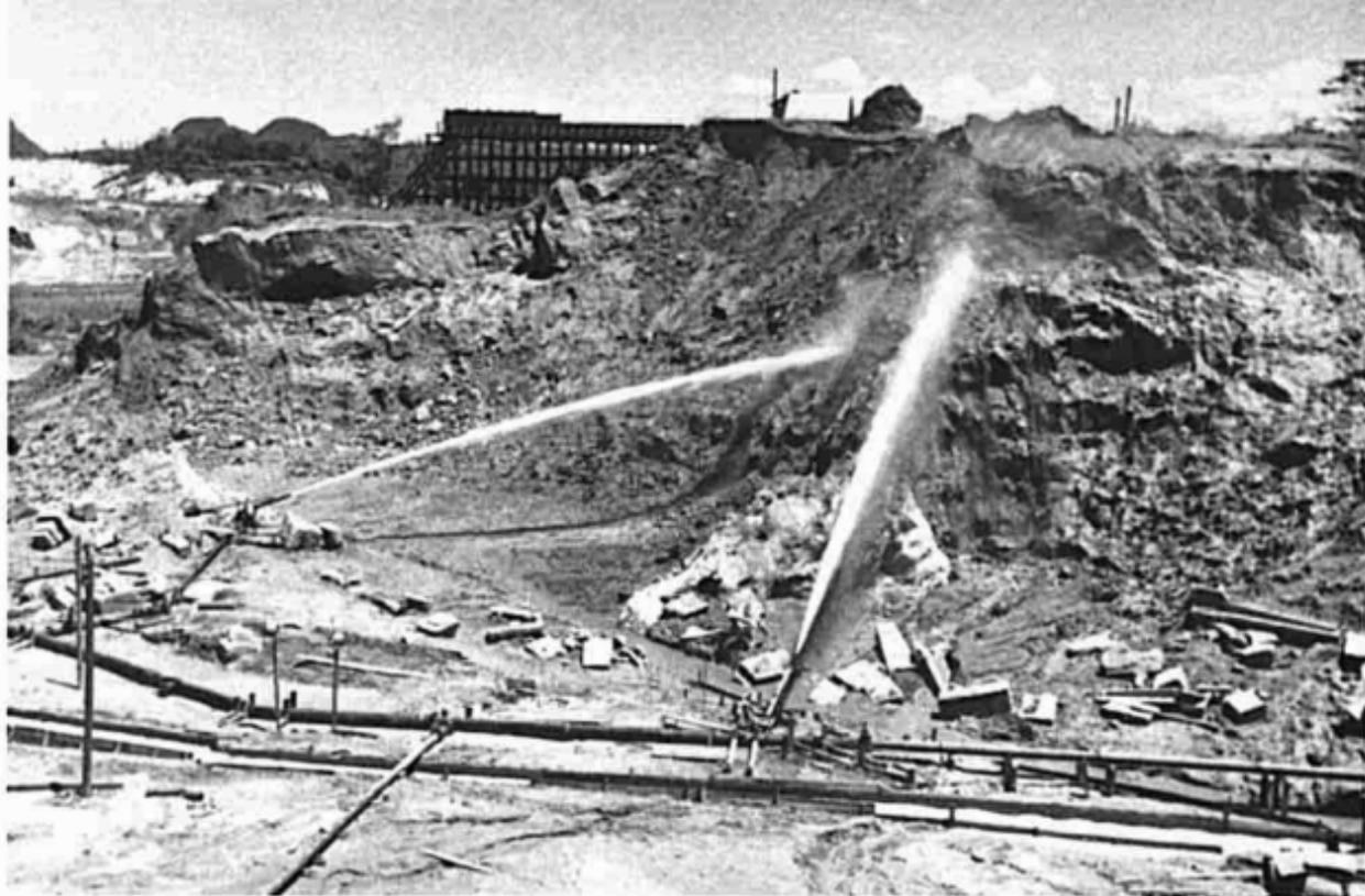
17. A Chinese-owned gravel-pump tin-mine. The tin-bearing earth is pounded by powerful water-jets. Note the 'palong', the raised wooden trough for washing down the tin-ore
