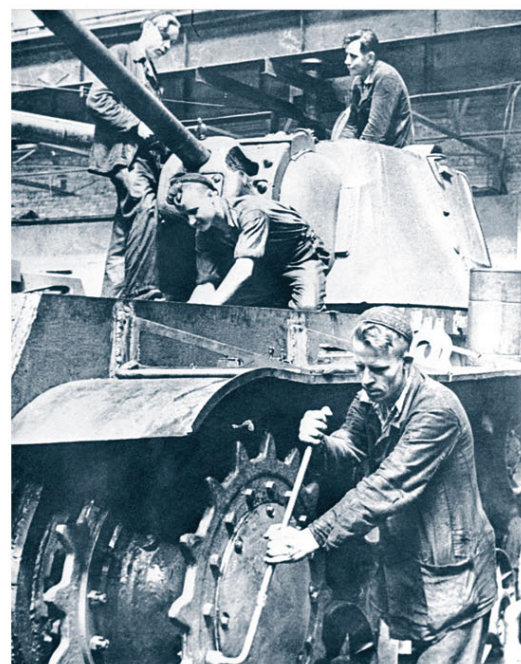
T-34 tank being assembled in Leningrad
