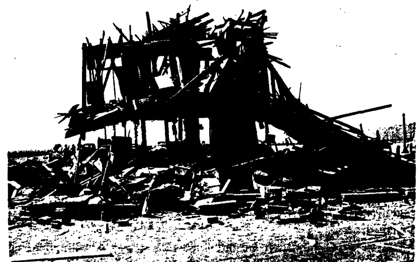
Figure 4.30. Unreinforced brick house after the nuclear explosion (5 psi overpressure).
