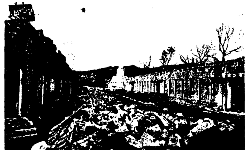
Figure 4.89a. Interior of two-story, brick wall-bearing building; the walls were 19 inches thick (0.80 mile from ground zero at Hiroshima). Blast collapsed the roof and second story and part of the first story, but much of the damage was due to fire.
