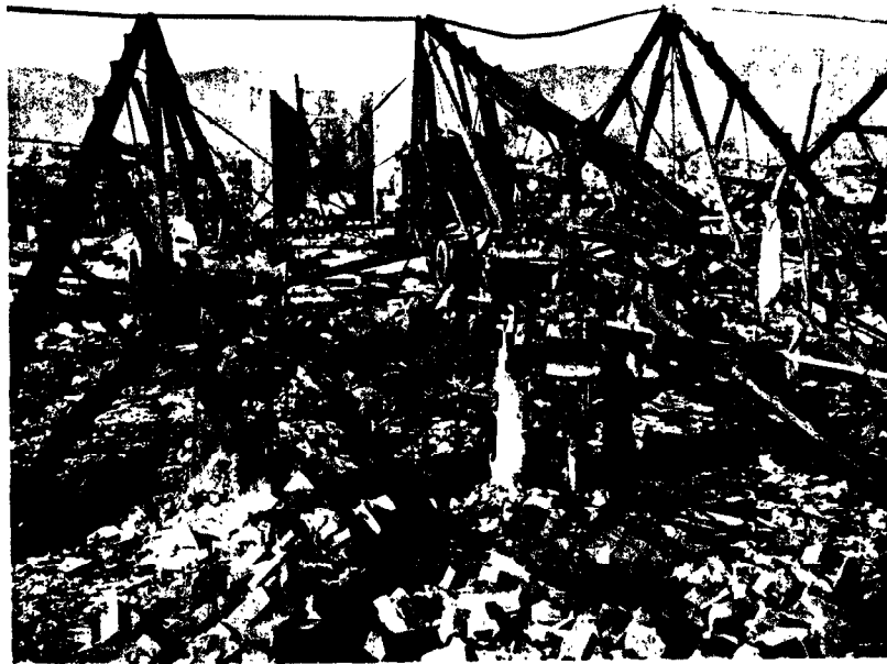
Figure 4.50. Damage to machine tools in steel-frame building (0.6 mile from ground zero at Hiroshima).
