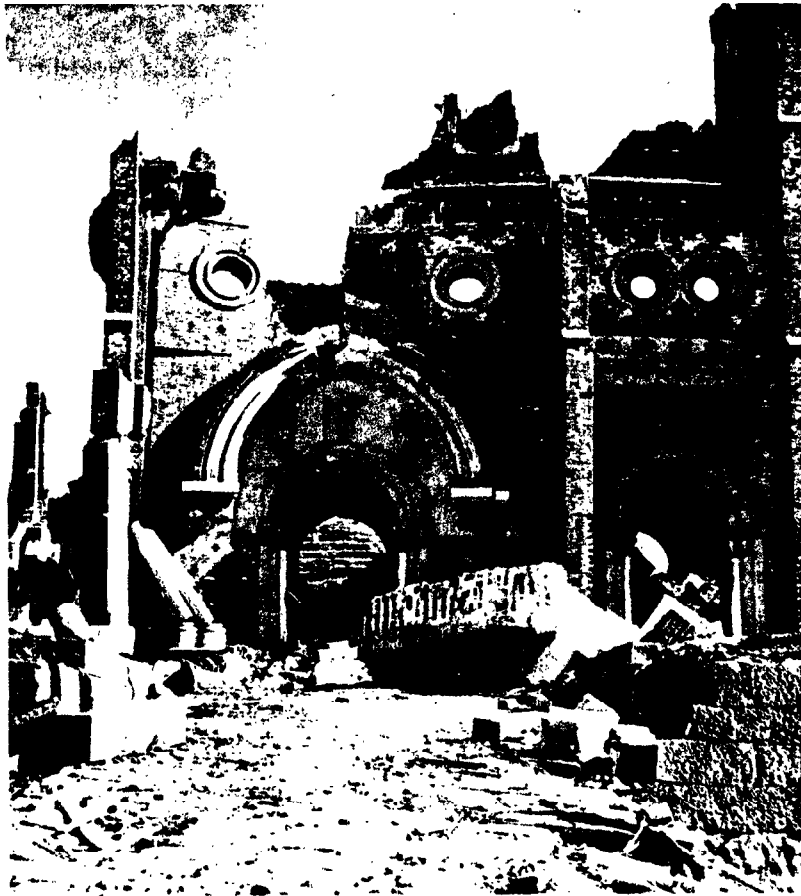
Figure 4.89b. Heavy wall-bearing structure; the 28-inch thick exterior walls of brick with buttresses were shattered (0.34 mile from ground zero at Nagasaki).
