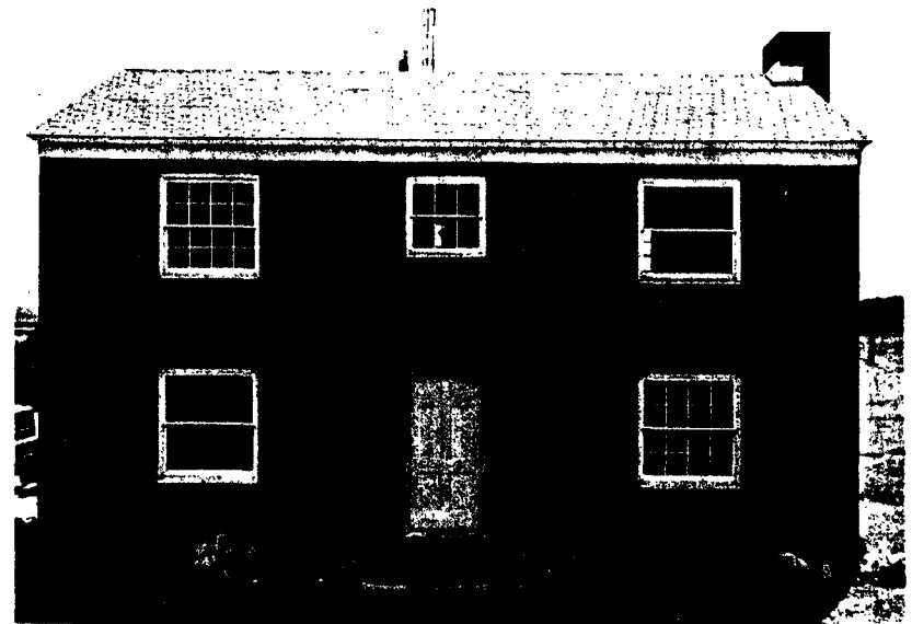
Figure 4.29. Unreinforced brick house before a nuclear explosion, Nevada Test Site.
