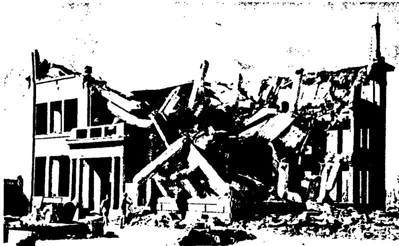
Figure 4.82b. Three story, reinforced-concrete frame building; walls were 13-inch thick brick panel with large window openings (0.13 mile from ground zero at Hiroshima).
