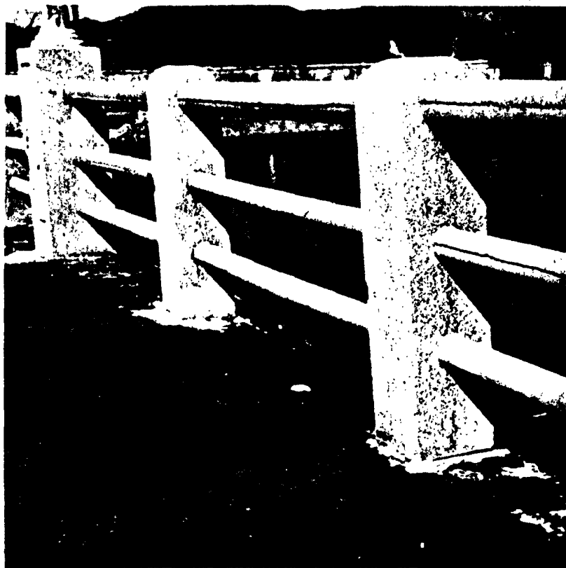
Figure 7.75a. Flash marks produced by thermal radiation on asphalt of bridge in Hiroshima. Where the railings served as a protection from the radiation, there were no marks; the length and direction of the "shadows" indicate the point of the bomb explosion.
