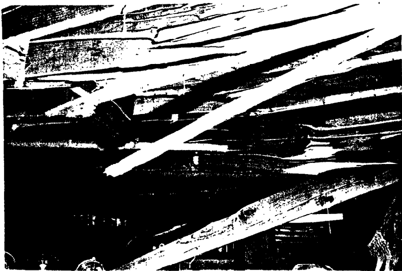
Figure 4.24 First floor joists of strengthened wood-frame house after a nuclear explosion (4 psi overpressure).
