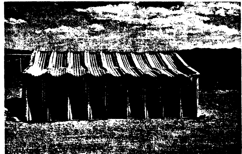
Figure 4.70. Self-framing corrugated steel panel building after the nuclear explosion (3.1 psi overpressure).
