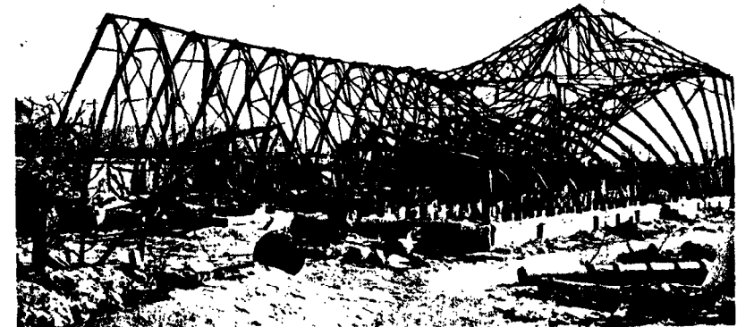
Figure 4.55b. Single story, light steel-frame building (0.8 mile from ground zero at Hiroshima); partially damaged by blast and further collapsed by subsequent fire.
