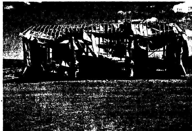
Figure 4.62b. Rigid steel-frame building after the nuclear explosion (3.1 psi overpressure).
