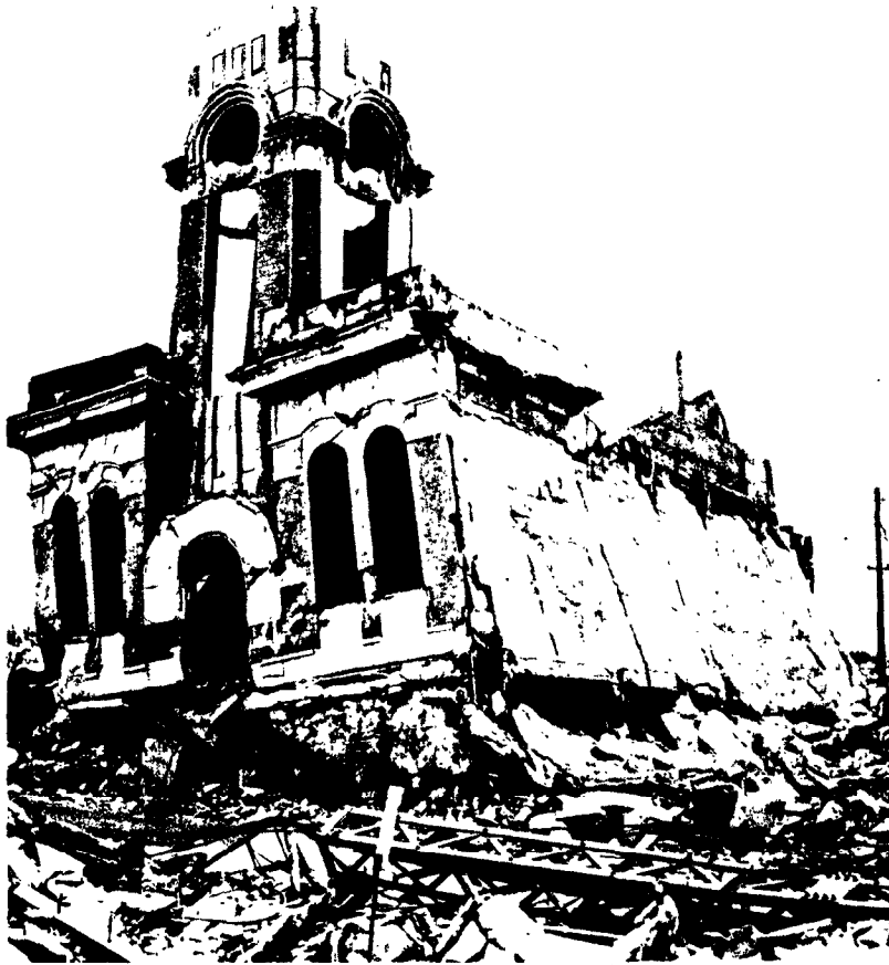
Figure 4.88 Two story steel-frame building with 7-inch reinforced-concrete wall panels (0.40 mile from ground zero at Hiroshima). The first story columns buckled away from ground zero dropping the second story to the ground.
