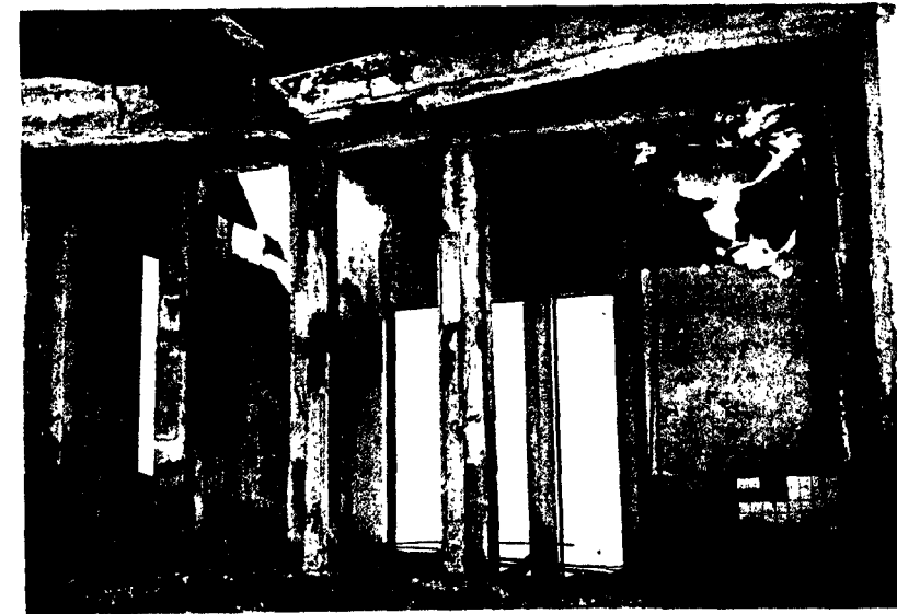
Figure 4.82a. Upper photo: Reinforced-concrete, aseismic structure; window fire shutters were blown in by blast and the interior gutted by fire (0.12 mile from ground zero at Hiroshima). Lower photo: Burned out interior of similar structure.
