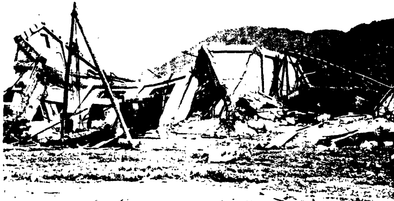
Figure 4.84c. One story, reinforced-concrete building with steel roof trusses (0.26 mile from ground zero at Nagasaki). Note the resistance offered by end interior walls when acting as shear walls.
