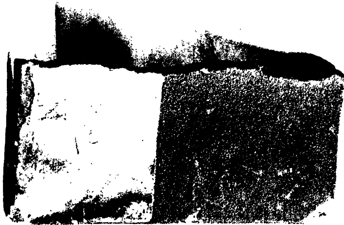
Figure 7.77. Blistered surface of roof tile; left portion of the tile was shielded by an overlapping one (0.37 mile from the explosion at Hiroshima).
