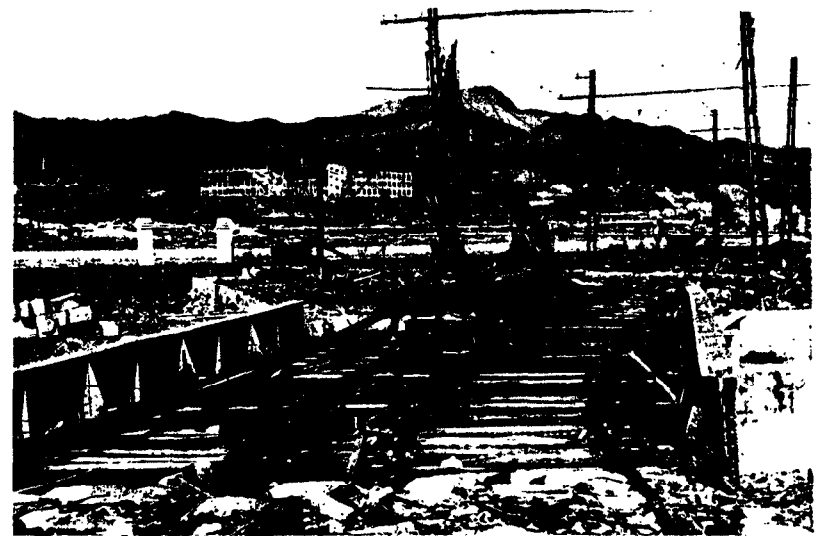
Figure 4.90b. A steel-plate girder, double-track railway bridge (0.16 mile from ground zero at Nagasaki). The plate girders were moved about 3 feet by the blast; the railroad tracks were bent out of shape and trolley cars were demolished, but the poles were left standing.
