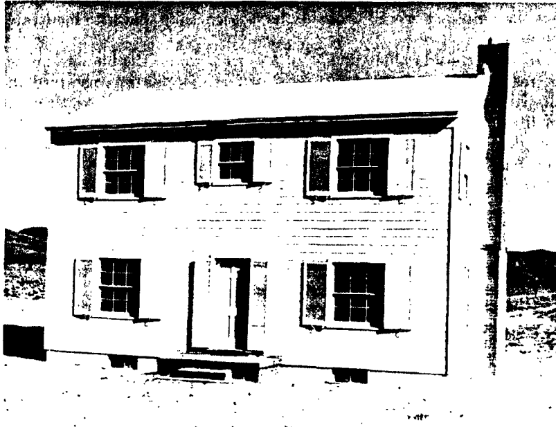
Figure 4.12 Wood-frame house before a nuclear explosion, Nevada Test Site.
