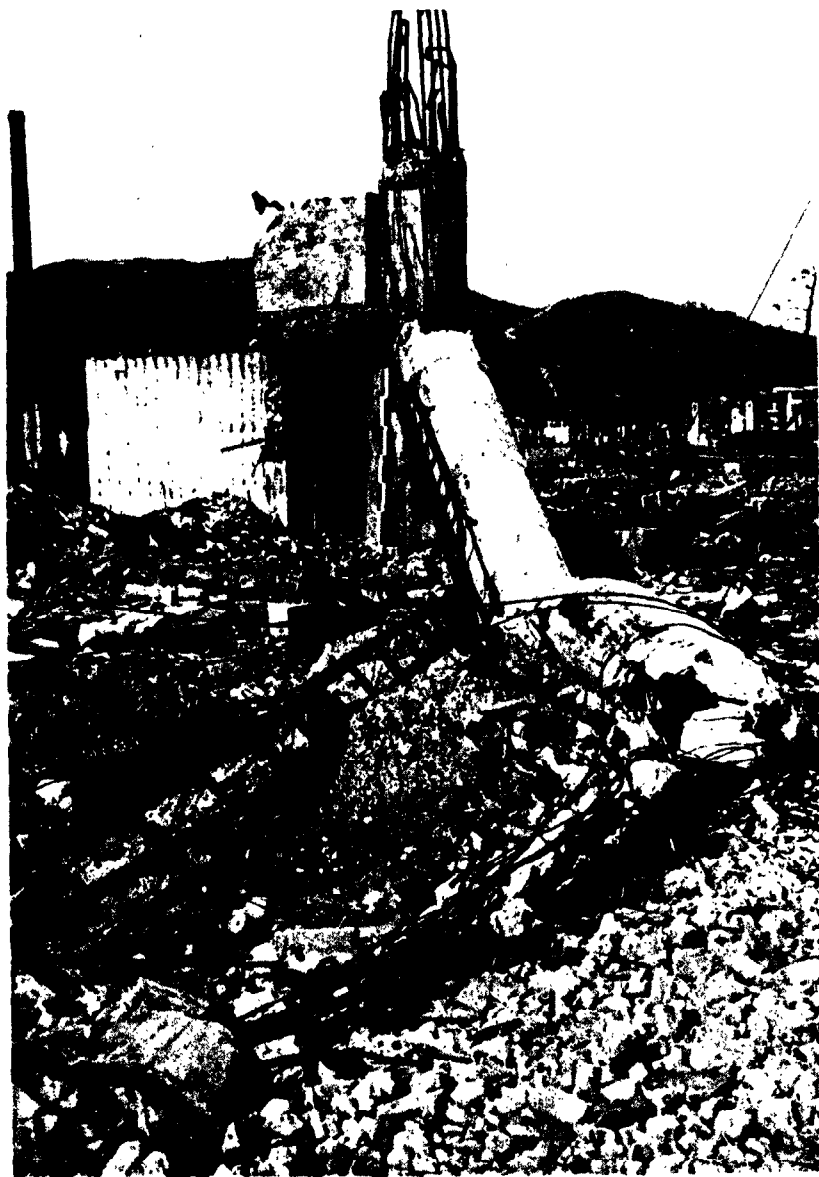
Figure 4.60b. A circular, 60 feet high, reinforced-concrete stack (0.34 mile from ground zero at Hiroshima). The failure caused by the blast wave occurred 15 feet above the base.
