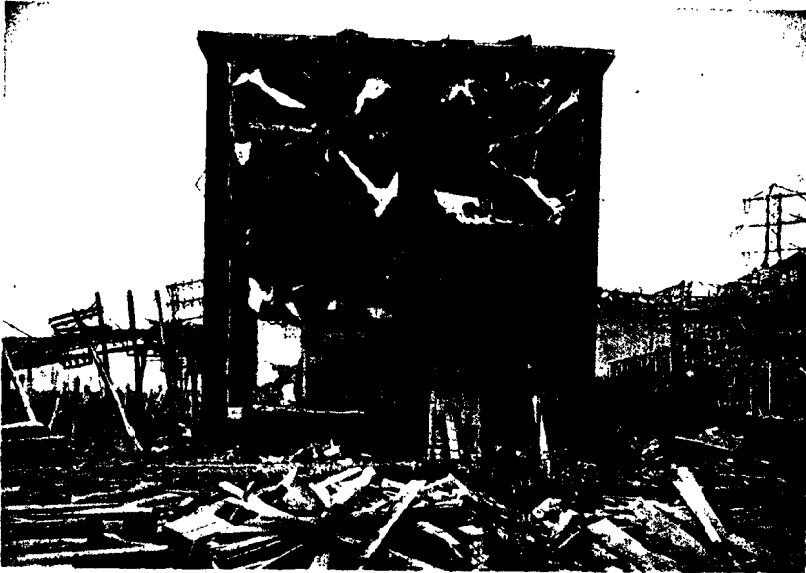
Figure 4.85c. Reinforced-concrete frame building showing crushed concrete panel walls on side facing explosion (0.68 mile from ground zero at Nagasaki).
