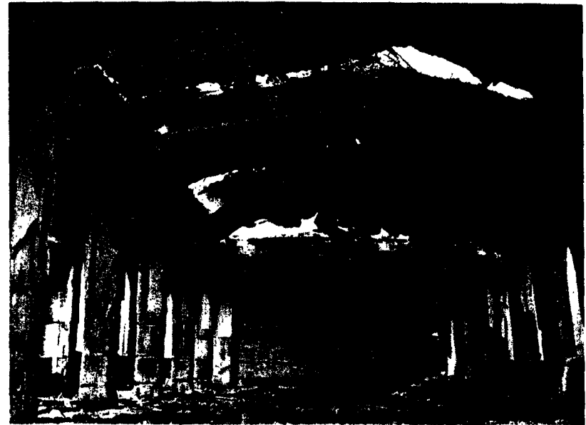
Figure 4.85a. Buckling and cracking of beams in reinforced-concrete building (0.32 mile from ground zero at Nagasaki).
