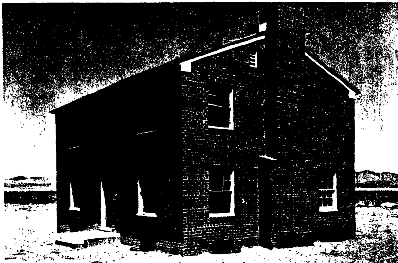
Figure 4.31. Unreinforced brick house after the nuclear explosion (1.7 psi overpressure).
