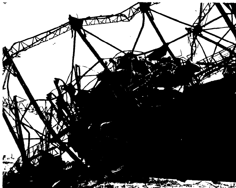
Figure 4.115. Gas holder destroyed by nuclear explosion (0.63 mile from ground zero at Nagasaki).
