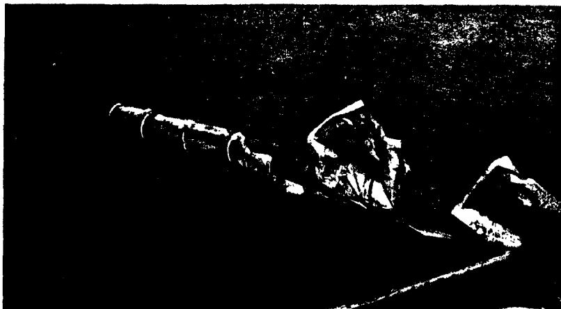
Figure 4.113b. Broken portion of 16-inch water main carried on bridge (0.23 mile from ground zero at Hiroshima).
