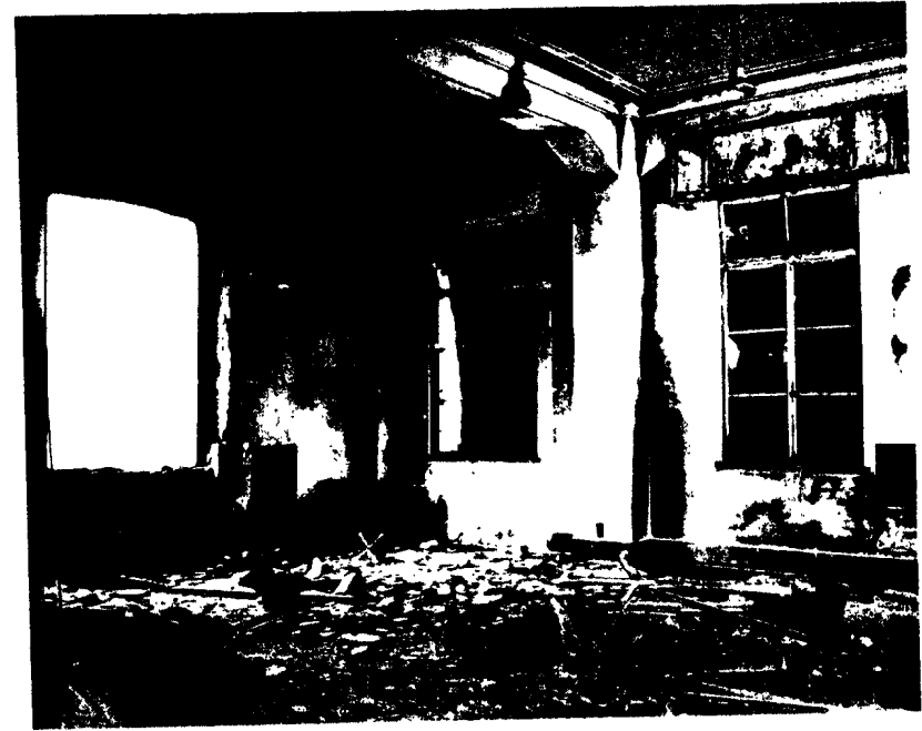
Figure 7.95. Fire shutters in building blown in or damaged by the blast; shutter at center probably blown outward by blast passing through building (0.57 mile from ground zero at Hiroshima).
