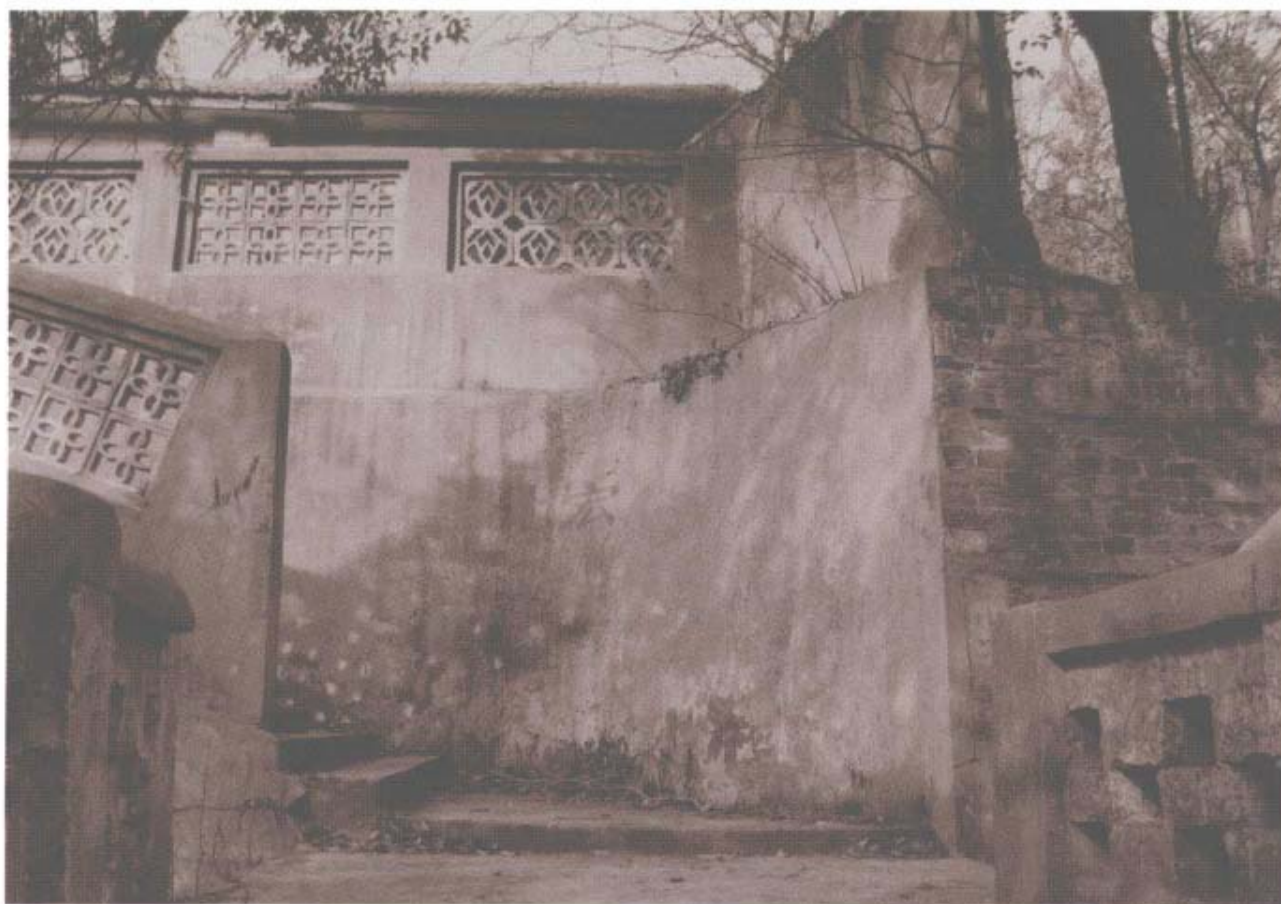
南京祖堂山精神病院旧址 (图2) Former Site of Nanjing Zutangshan Mental Hospital (Picture 2)
