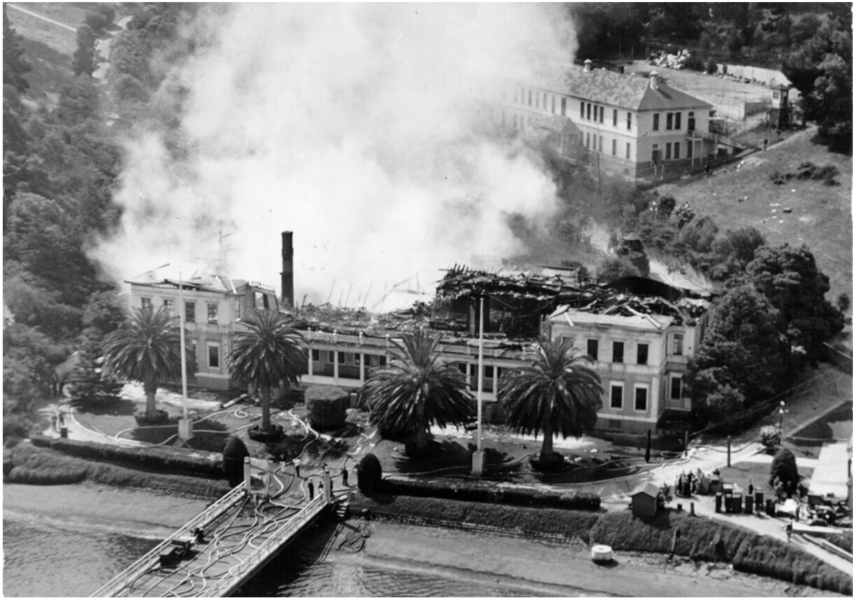
At midnight on August 12, 1940, a fire broke out. Caused by an overloaded circuit in the basement of the administration building, it almost led to the total destruction of the immigration station. Bellows of smoke rising over the administration building could be seen the next morning after firefighters battled through the night to contain the fire. (San Francisco History Center, San Francisco Public Library.)
