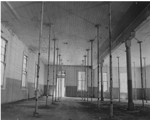
Room 105, the Chinese men's barracks on the first floor of the detention building, 1970s. Each pole could hold three tiers of bunk beds on each side. (Photo by Chris K. D. Huie.)
