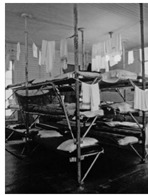
Refurbished women's quarters in the detention building, 1980s. (Photo by Daniel Quan.)
