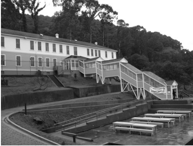
Restored detention barracks with covered stairway and tables where the dining room once stood, 2009. (Photo by Vincent Chin.)
