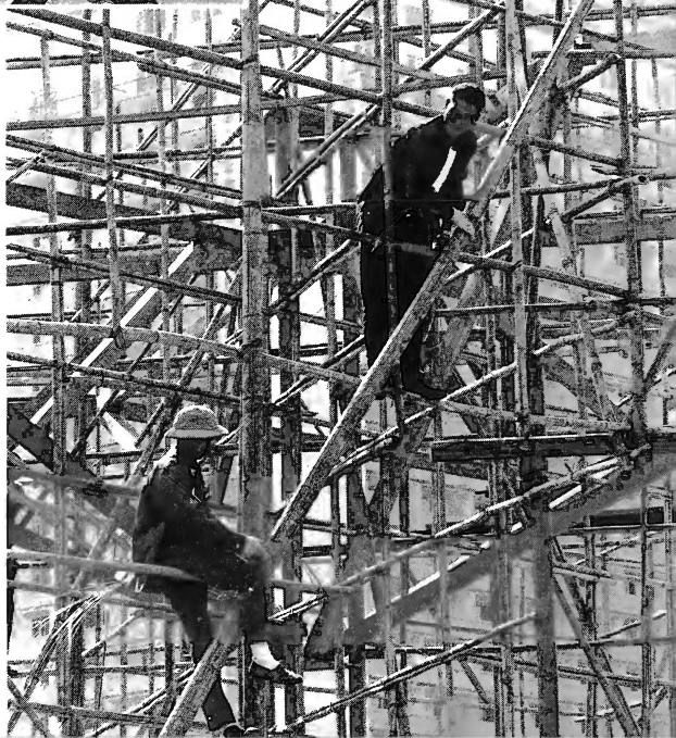
RIGHT: Bamboo scaffolding is used for high-rise building. This intricate network has the Mandarin Hotel as a background.
