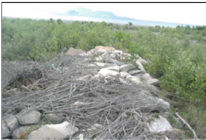
(a) Groyne exposed after December 2004 tsunami with wide mangrove belt in front
