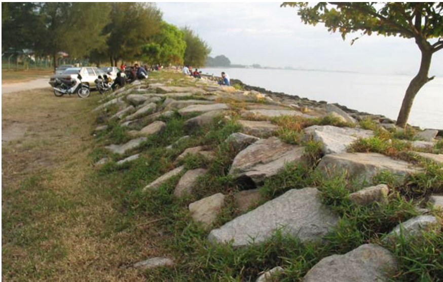
Fig. 5.13 Massive rock bund along Robina coast helped to mitigate the 2004 tsunami effects. Photograph taken five days after tsunami on 3 December 2004
