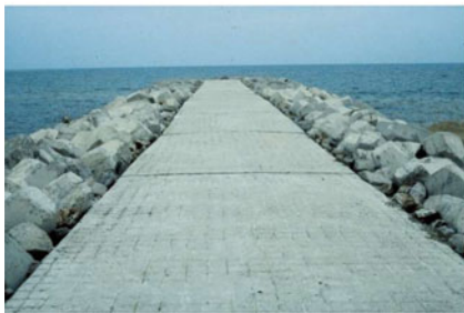
(c) Dungun groynes of concrete spine and tetrapods
