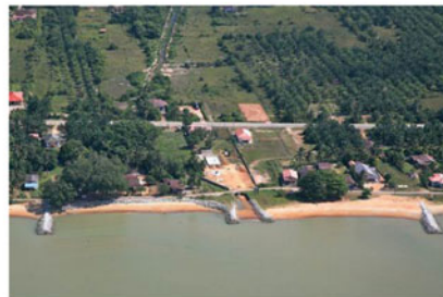
(d) Groyne and river mouth training wall of North Melaka
