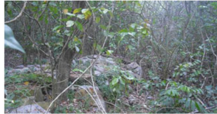
(b) Groyne 2 hidden under coastal bushes-2012 September
