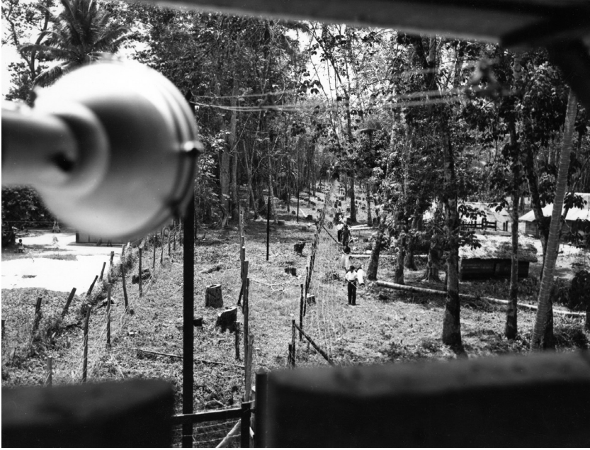
Figure 8. The view from one of the fifteen watchtowers surrounding the New Village of Tanjong Malim, northwest Malaysia (undated, likely early 1950s). British authorities forcibly relocated half a million Malayan Chinese into such New Villages to cut them off from the MCP. Photo courtesy of the Imperial War Museums.
