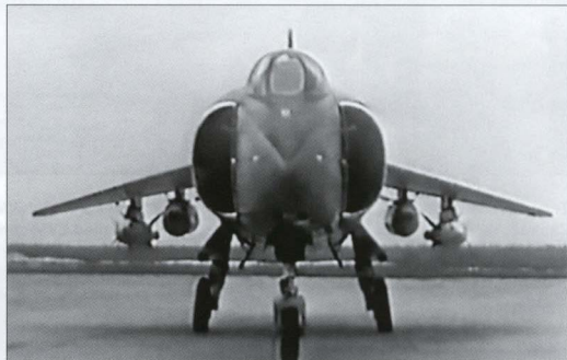
Above and with: '01 Yellow', the izdeliye EVM full-size presentation mock-up of the Yak-36M shows off the short nose, strong wing and tailplane anhedral, horizontally clipped fin tip and narrow landing gear track. There are no recirculation dams yet.
