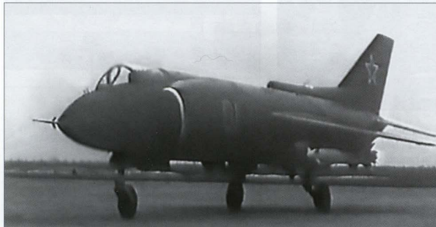
Above and with: '01 Yellow', the izdeliye EVM full-size presentation mock-up of the Yak-36M shows off the short nose, strong wing and tailplane anhedral, horizontally clipped fin tip and narrow landing gear track. There are no recirculation dams yet.
