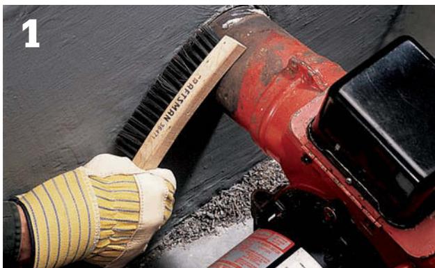
Use a wire brush to clean off any rust or dirt deposits that have accumulated on the surface.
