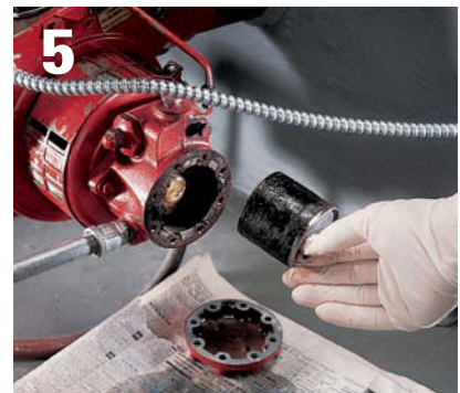
5 Remove the mesh strainer carefully. Even a heavily soiled one can often be reused after a good cleaning.
