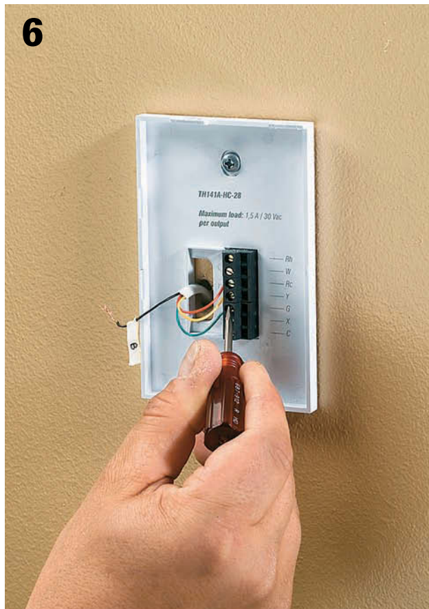
6 Check the manufacturer's instructions to establish the correct terminal for each low-voltage wire. Then connect the wires to these terminals, making sure each screw is secure.
