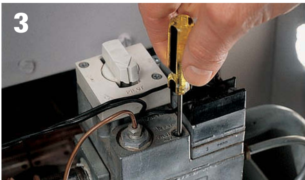
3 Turn the screw to adjust the height of the flame so it covers the top of the thermocouple.
