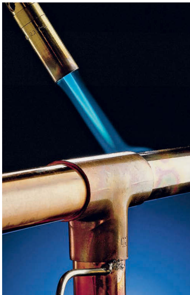
Soldered fittings , also called sweat fittings, often are used to join copper pipes. Correctly soldered fittings are strong and trouble-free. Copper pipe can also be joined with compression fittings or flare fittings. See chart below.
