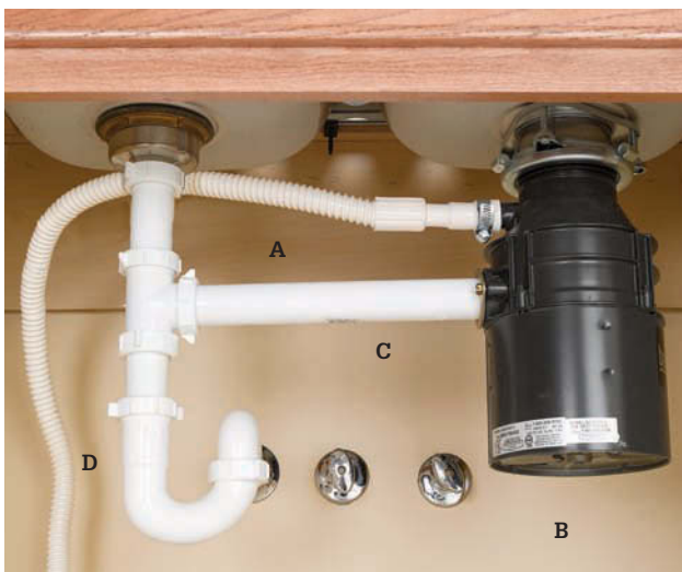
In this arrangement, the dishwasher drain hose (A) attaches to the food disposer (B), and a trap arm (C) leads from the disposer to the P-trap (D).
