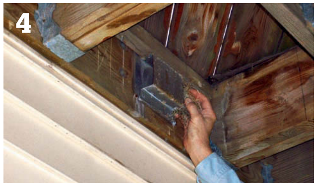
4 Remove any debris and materials that could block the air intake and exhaust.
