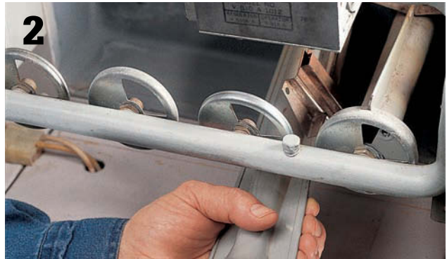
2 If a burner is difficult to remove, twist it carefully from side to side while lifting and pulling.
