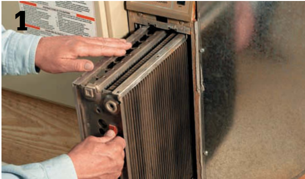
1 Clean electronic filters every month, then reinsert them in your furnace.
