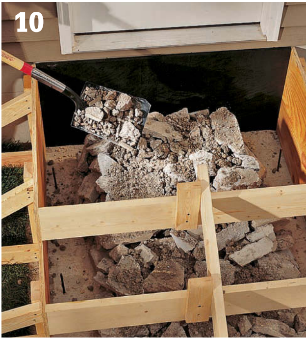
10 Fill the form with clean fill (broken concrete or rubble). Stack the fill carefully, keeping it 6" away from the sides, back, and top edges of the form. Shovel smaller fragments onto the pile to fill the void areas.
