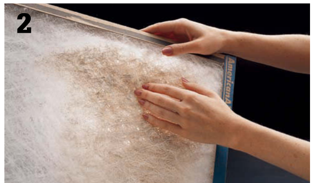
Hold the filter up to a bright light for inspection.
