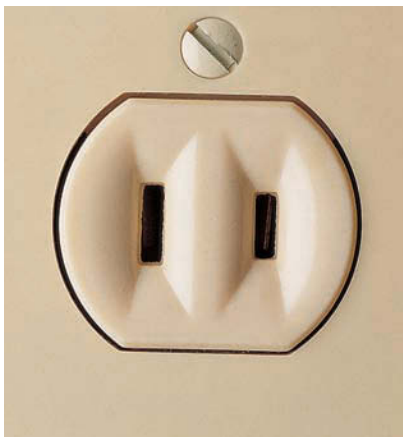
15 amps, 120 volts. Polarized two-slot receptacles are common in homes built before 1960. Slots are different sizes to accept polarized plugs.
