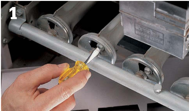
1 Remove the screws holding the burners to their brackets or to a slide-out pan.
