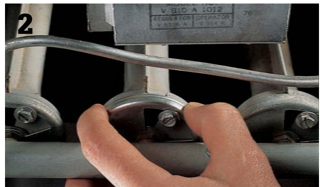
2 If the shutters are adjustable, you can set them yourself. Otherwise, call a professional for service.
