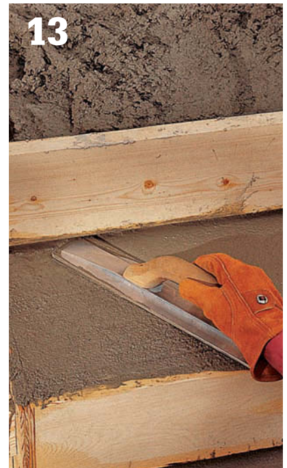
13 Float the steps , working the front edge of the float underneath the beveled edge at the bottom of each riser form.
