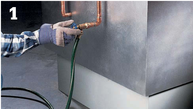
Use a garden hose to drain water from the boiler. Keep the drain end of the hose lower than the drain cock on the boiler.
