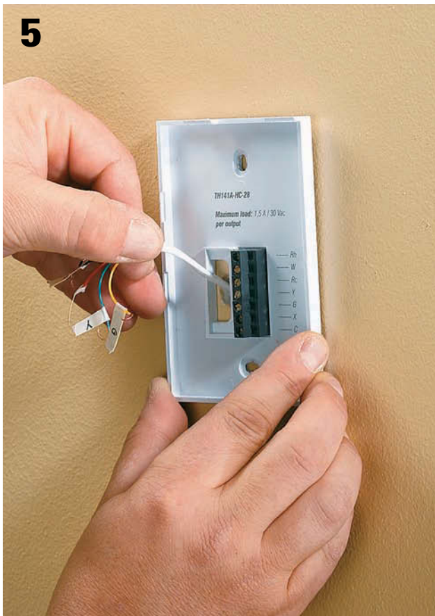
5 Position the new thermostat base on the wall, and guide the wires through the central opening. Screw the base to the wall using wall anchors if necessary.
