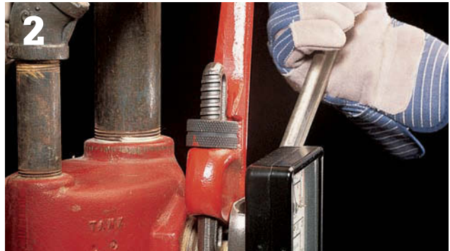
If the valve or gauge on top of the boiler is attached to a separate fitting, hold the fitting still with one wrench while removing the valve or gauge with another.
