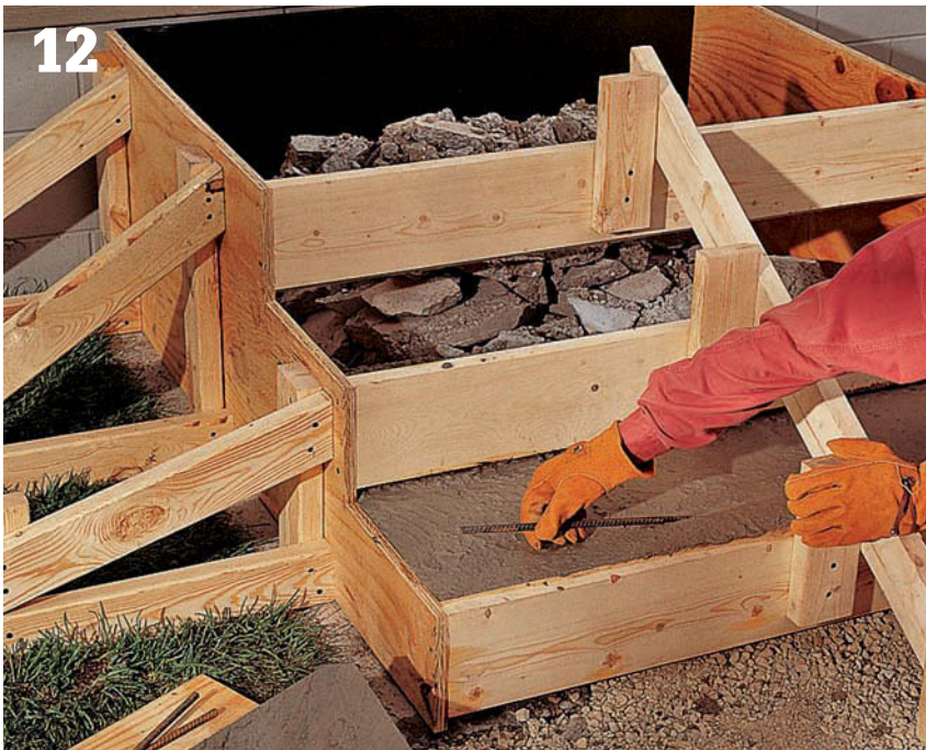
12 Coat the forms with vegetable oil or a commercial release agent , then mist them with water so concrete won't stick to the forms. Mix concrete and pour steps one at a time, beginning at the bottom. Settle and smooth the concrete with a screed board. Press a piece of #3 rebar 1" down into the "nose" of each tread for reinforcement.
