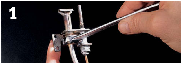
1 Loosen the connecting nut on the gas line with an open-end wrench.
