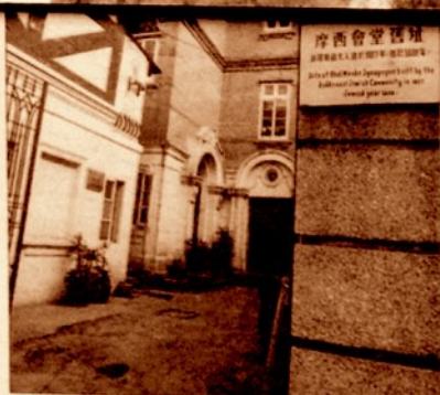
Ohel Moishe Synagogue, 62 Changyang Road in Hongkou District.
