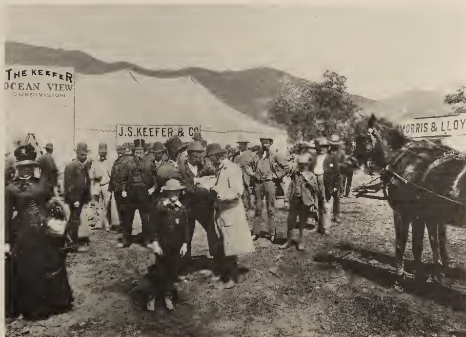
The auction opening the Myrtle Avenue subdivision in Monrovia—and the ocean was very far away, ca. 1887.
