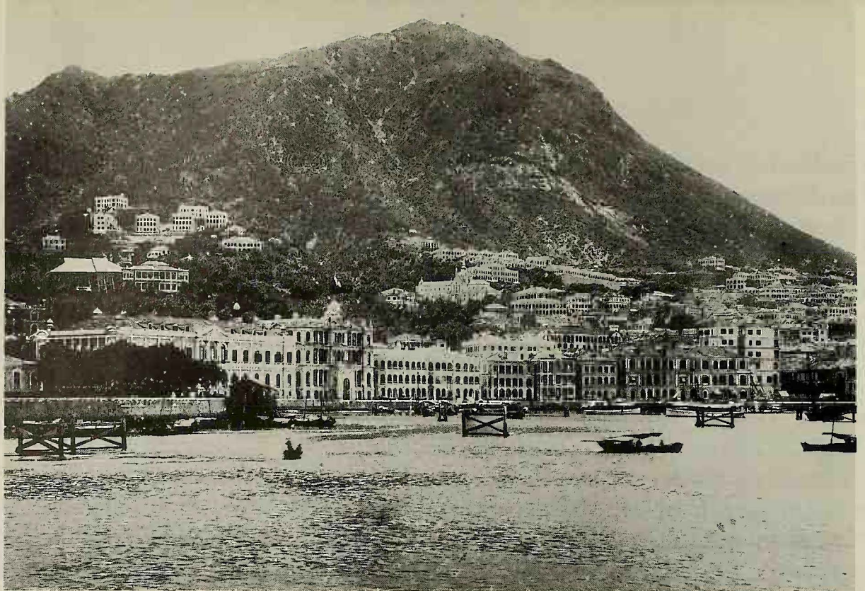
The Praya before reclamation. Markers in the harbour show the extent of the new land to be formed. Wardley House, the Hongkong and Shanghai Bank's second building, is the domed structure just left of centre with the City Hall on its left.
