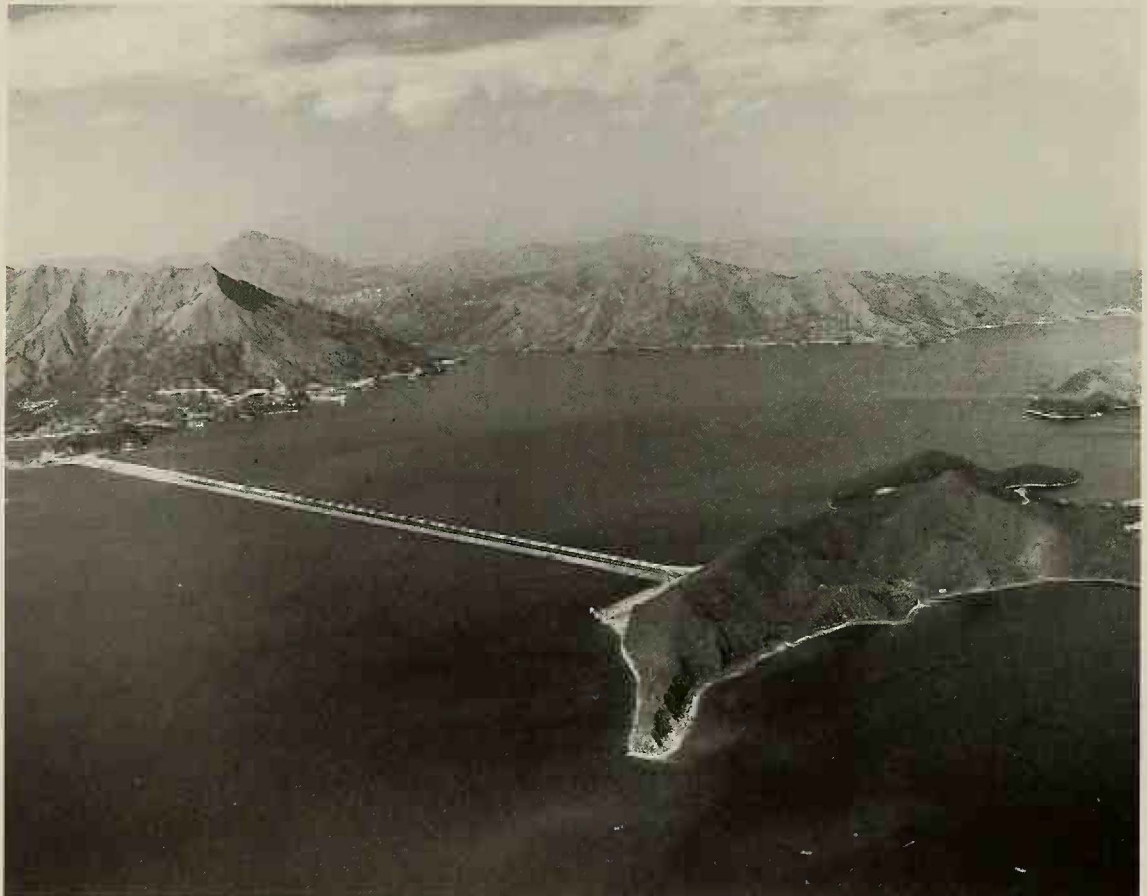
The first of the new reservoirs constructed to supply the needs of a rapidly rising population and growing industry was formed at Plover Cove in 1968.
