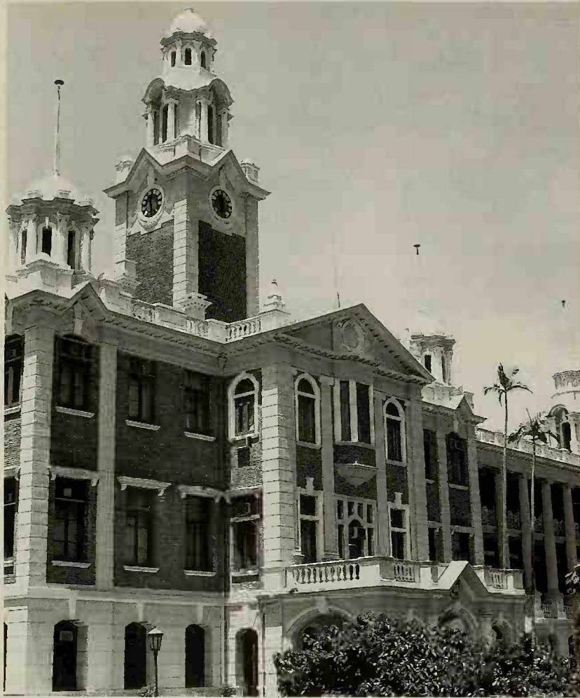
The façade of the original buildings of Hong Kong University.
