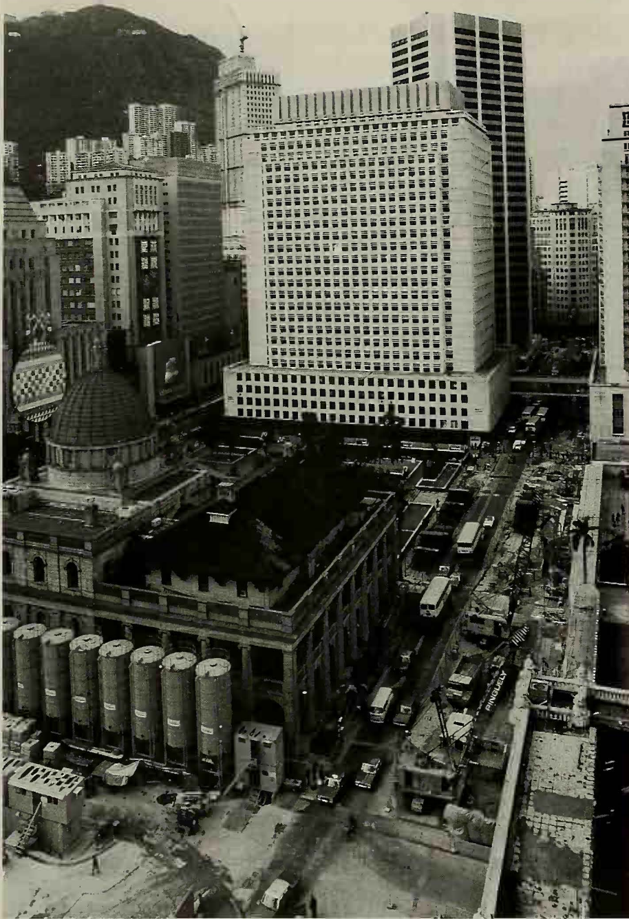
The construction of the Mass Transit Railway, Hong Kong's Underground or Metro, disrupted life for some time.
