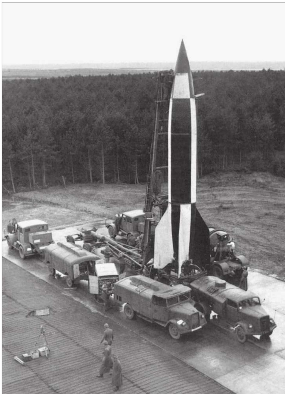
A V-2 is prepared for a test launch by a German crew under the British-organised Operation Backfire programme. Bill Rose
