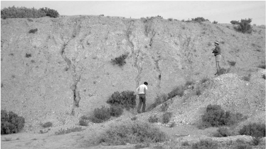
Fig.2. Rill erosion of the soil capped tailings storage facility, Radium Hill, South Australia (height of facility approximately 6 m). The soil capping is being removed, resulting in the exposure of radioactive tailings in rills.
