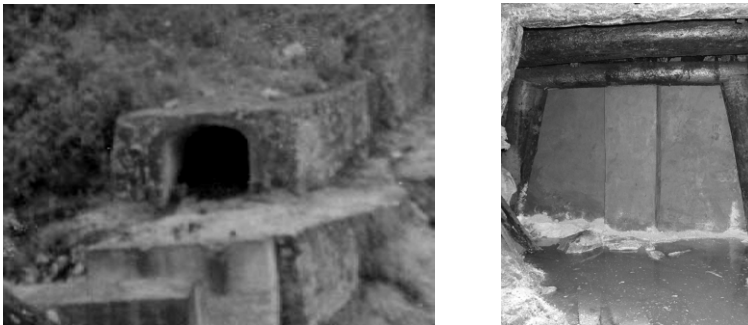
Fig.7. The inclined shaft before and during closure
