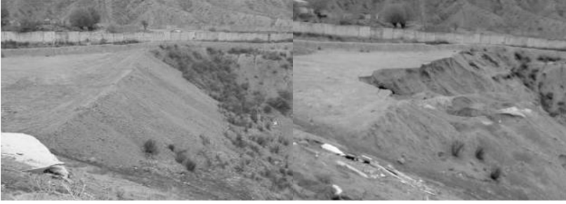
Fig.7. Tailings pile dam and cover built at Kadji-Say 2006 and state of the pile 2007
