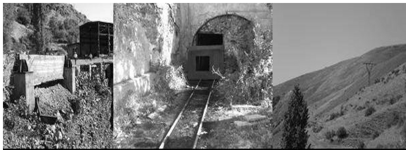
Fig. 4. Open mine adit and extensive uncovered waste rock piles at the Yanghiabad site.
