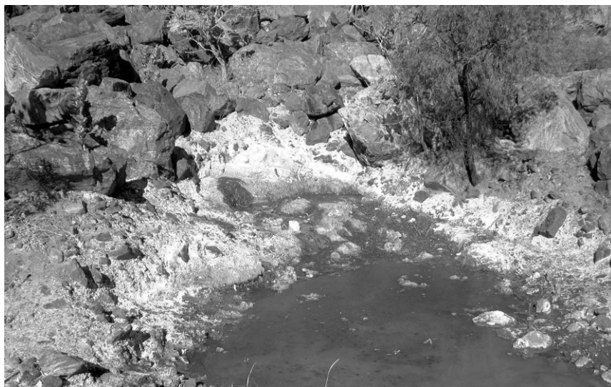
Fig. 3. Seepage point at the base of the tailings dam wall, Mary Kathleen, Australia. Abundant sulfate efflorescences and Fe-oxyhydroxide precipitates form from the acid, saline, radioactive seepage water (pH: 5.5; salinity: 0.31 %). Boulders in the retaining wall are approximately 1 m in diameter.
