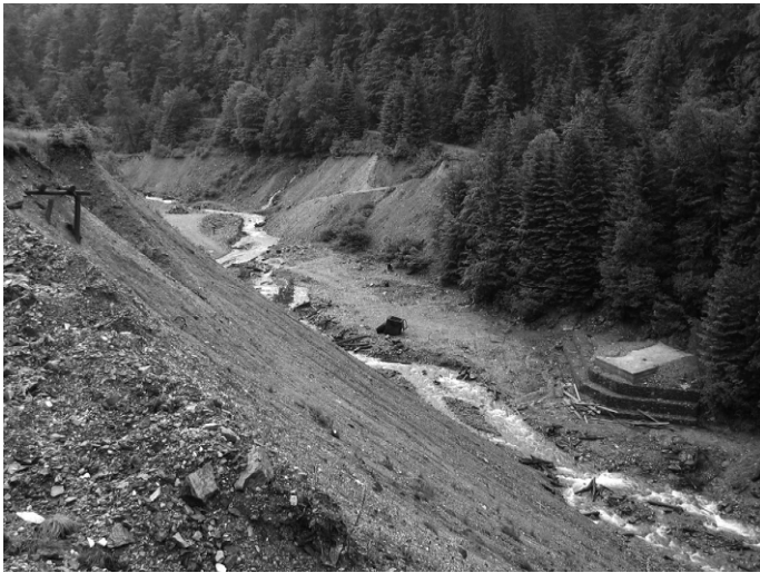
Fig.2. Waste dumps along Ariesul Mic river with pregnant erosional phenomena. On the left bank it may be seen the concrete seal of Aries Shaft.
