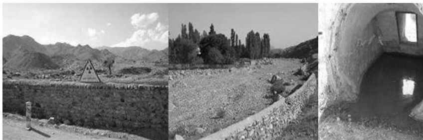
Fig. 5. The Charkesar-2 legacy site behind the wall, Charkesar village on the left bank of the river and mine water overflow from a ventilation shaft.
