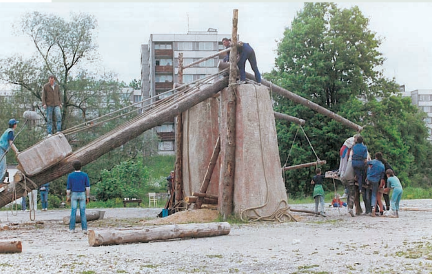
8.11–12 Reconstruction (above and below) of a possible method used to lift the lintel stones of the trilithons at Stonehenge.
