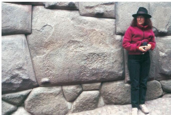
8.14–15 Inca stonework. (Right) The famous 12-angled stone in Cuzco, Peru, part of a wall of accurately fitted blocks built by the Incas. (Above) Diagrams illustrating Jean-Pierre Protzen's experiments to discover how Inca stonemasons may have dressed the blocks. Initially (left) Protzen pounded one face of the stone with a 4-kg (9-lb) hammer, which he twisted at the last minute to deliver a glancing blow. Then (center) he used a smaller 560-g (1.2-lb) hammer to prepare the edges of the next face. Having repeated the process for each face, he finally produced a finished block (right) with slightly convex corners, similar to the corners on actual Inca stonework.
