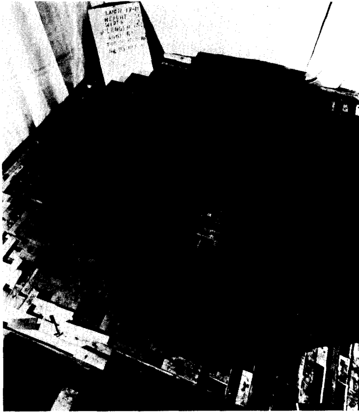
53. Chicago Pile Number One, the first man-made nuclear reactor, under construction at the University of Chicago, November 1942. Lower layer holds uranium oxide pseudospheres, unfinished dead layer overlying. Note hammer in foreground for scale.
