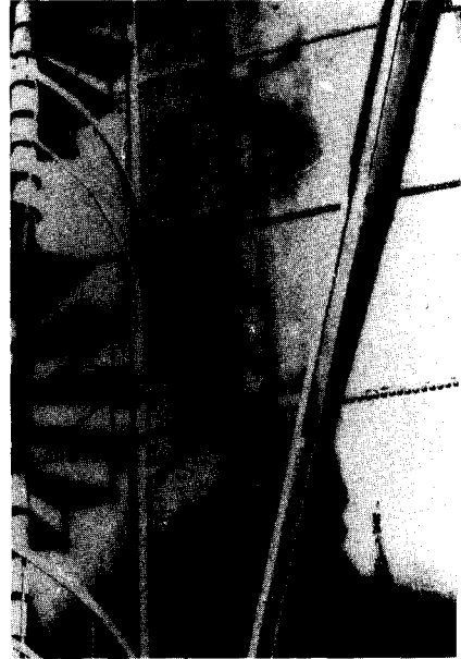
112. Staircase on a gas storage tank shadowed in uncharred paint, Hiroshima.
