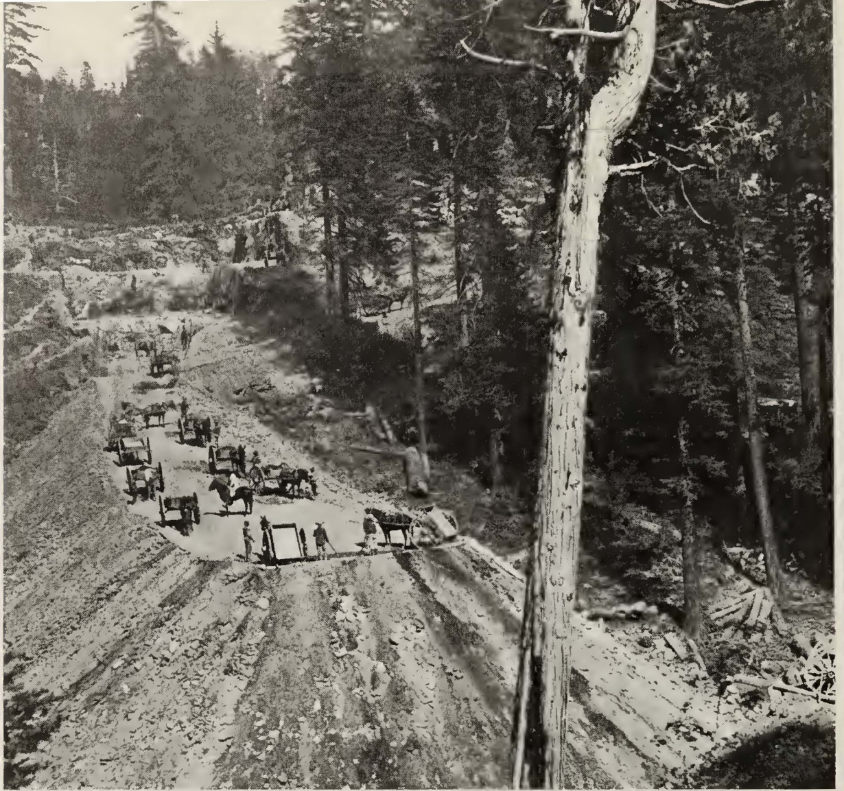
Crossing the Sierra required enormous fills, like this at Sailor's Spur. . .
