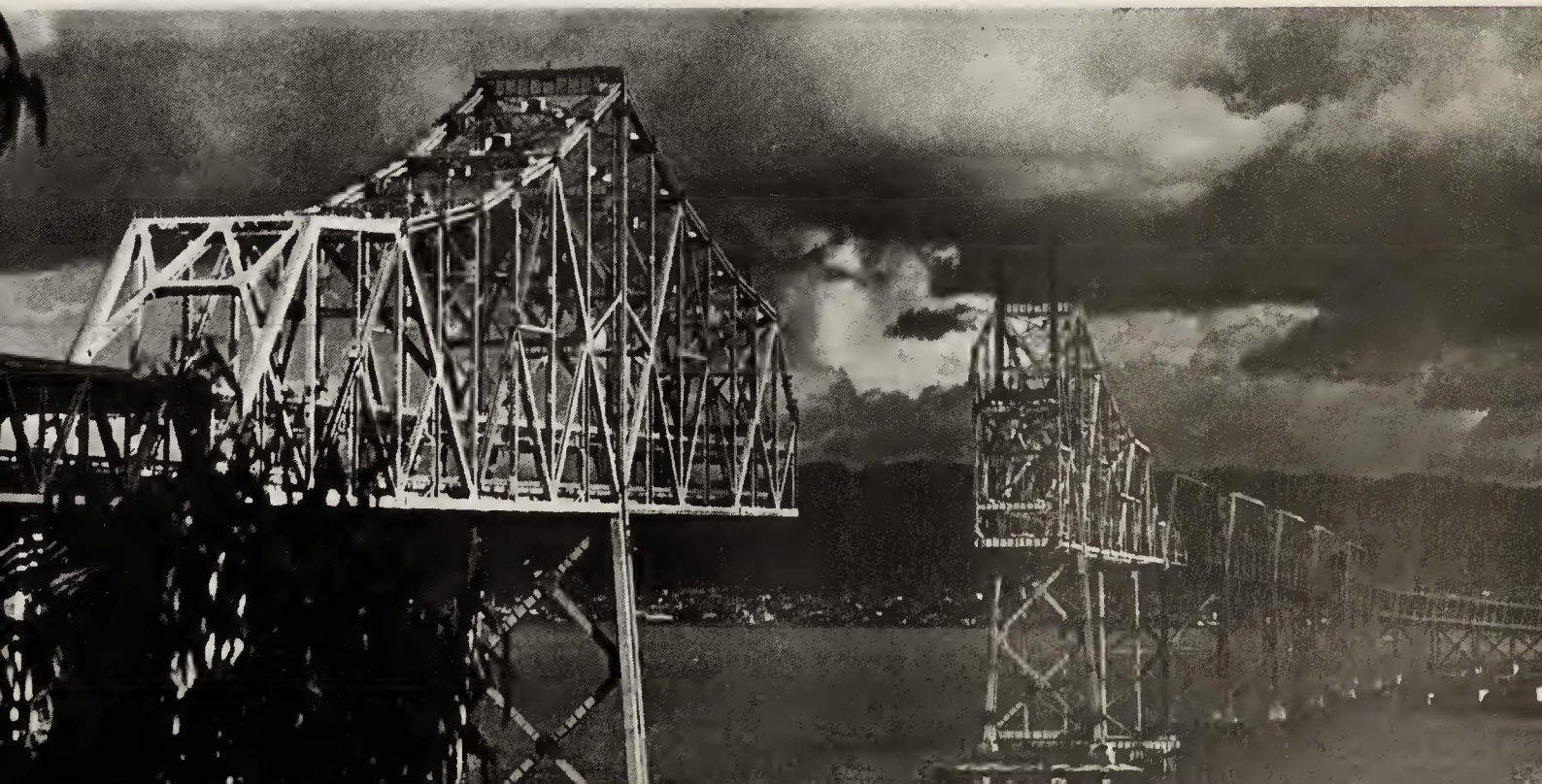
Like creatures out of H. G. Wells’ The War of the Worlds, the two ends of the Bay Bridge’s cantilever section prepare to meet.
