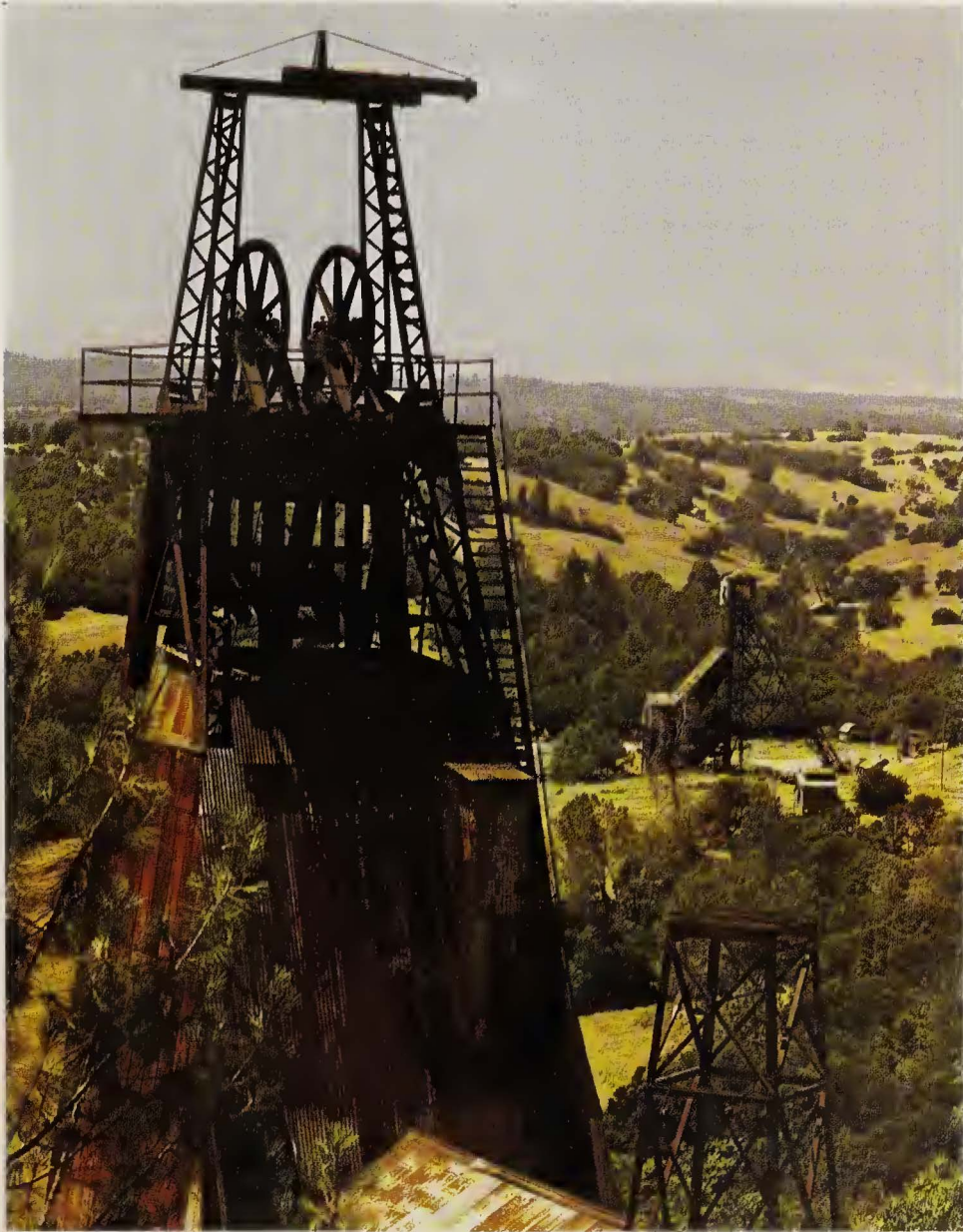
Headframe and hoisting shed of the Kennedy Mine, Jackson.
