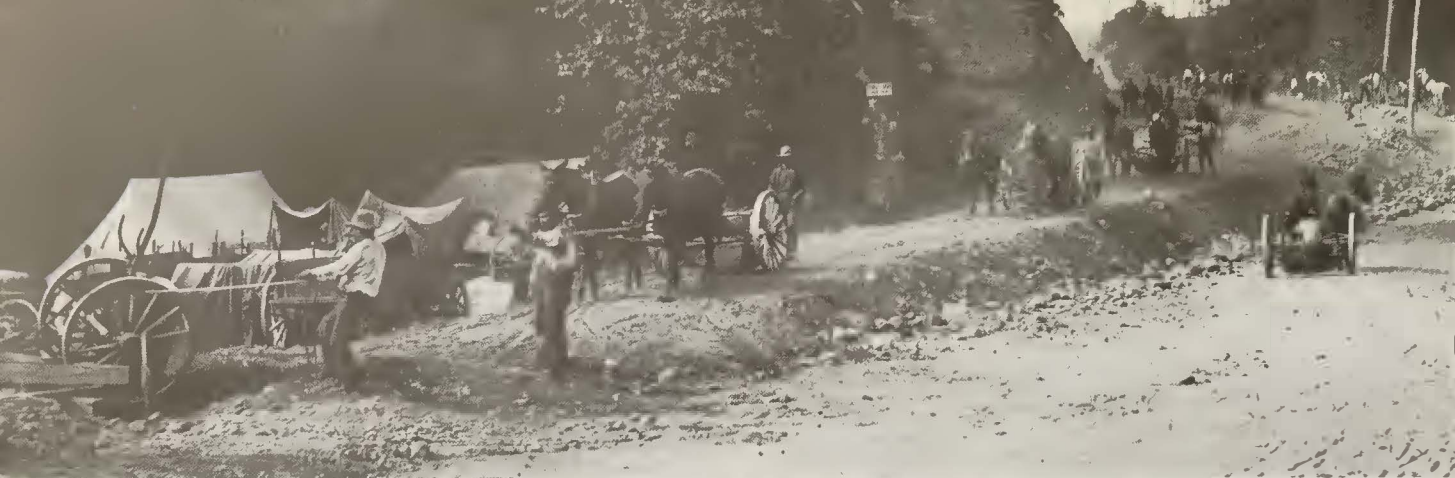
A study in contrasts: highway-building with horse-drawn Fresno scrapers.
