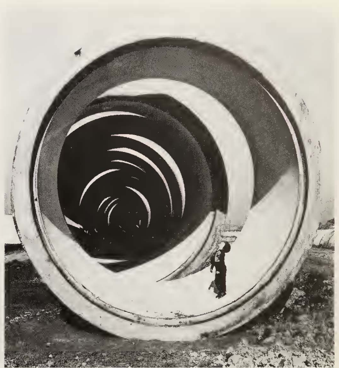
Prefabricated concrete pipe to carry water pumped from Tracy to the Delta-Mendota Canal, C. V. P.
