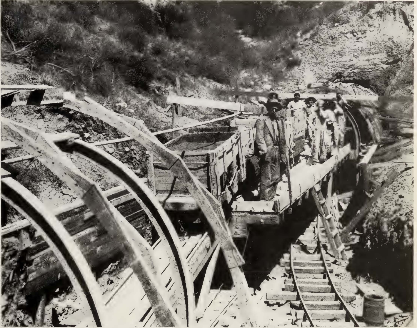
A crew of "muckers" poses outside one of the 142 tunnels drilled and lined with pipe during the construction of the 250-mile aqueduct.
