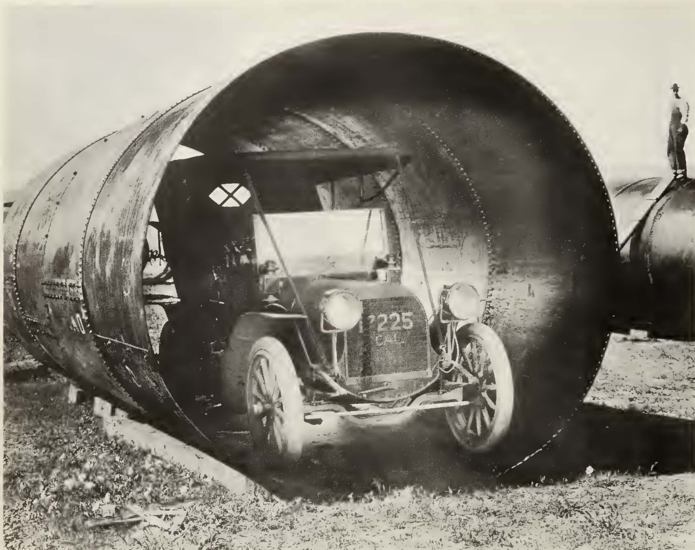
A Model T Ford demonstrates the size of the pipes used in the construction of the aqueduct's immense siphons.
