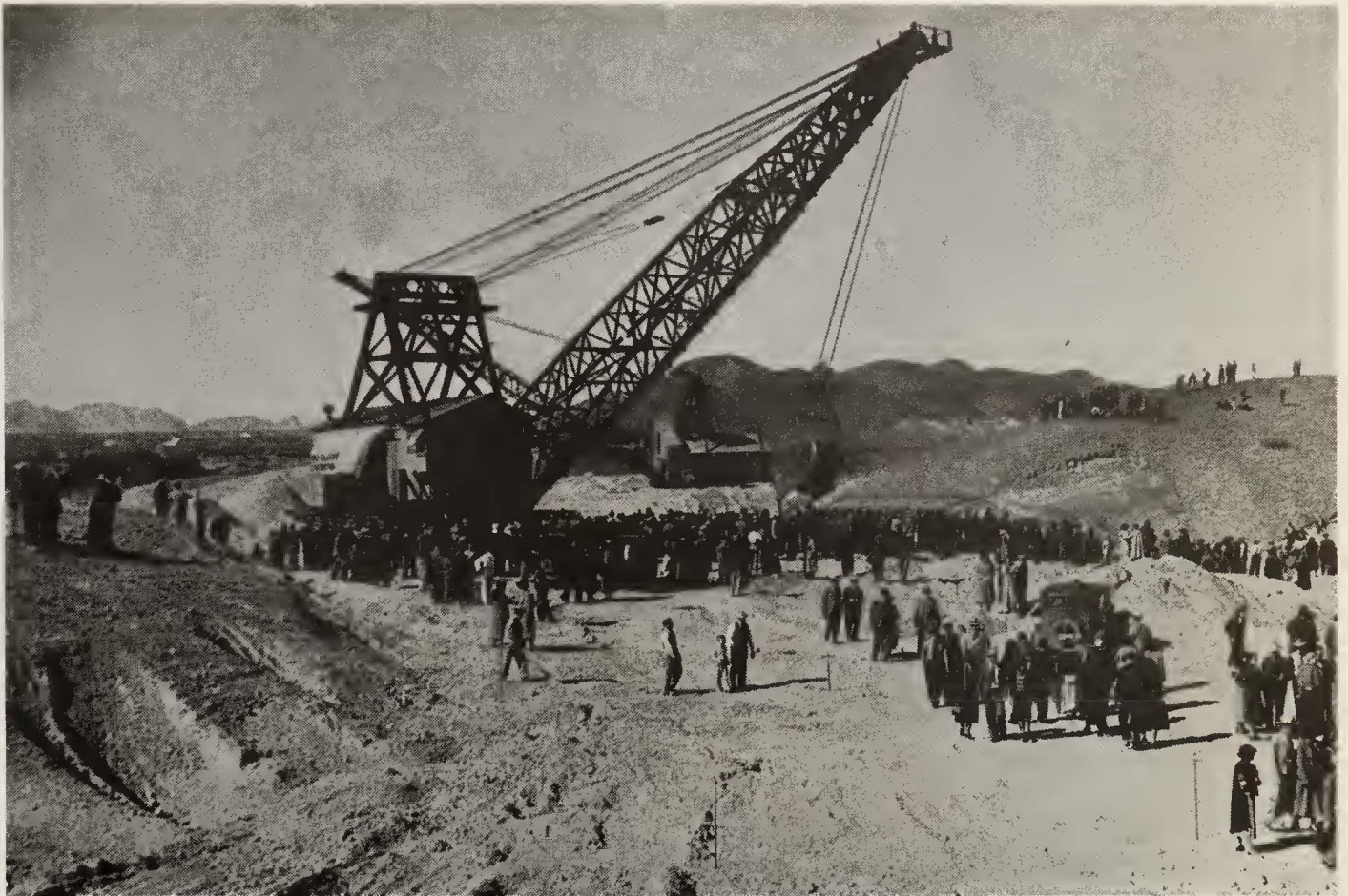
Construction on the route of the All-American Canal. The walking-bridge dredge shown above was first used on the Panama Canal.
