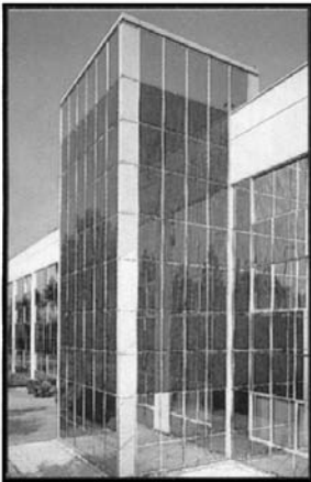
FIGURE 3-11 Building-integrated pv systems in Germany. (Source: Professional Engineering, Publication of the Institution of Mechanical Engineers, April 1997, U.K.. With permission.)
