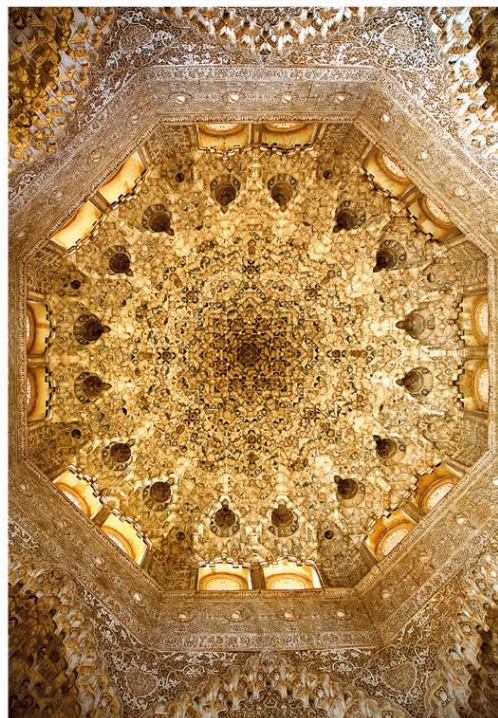
Ceiling of the Hall of the Two Sisters: this worm’s-eye view of the interior of its muqarnas dome shows its cell-like patterning in stucco
