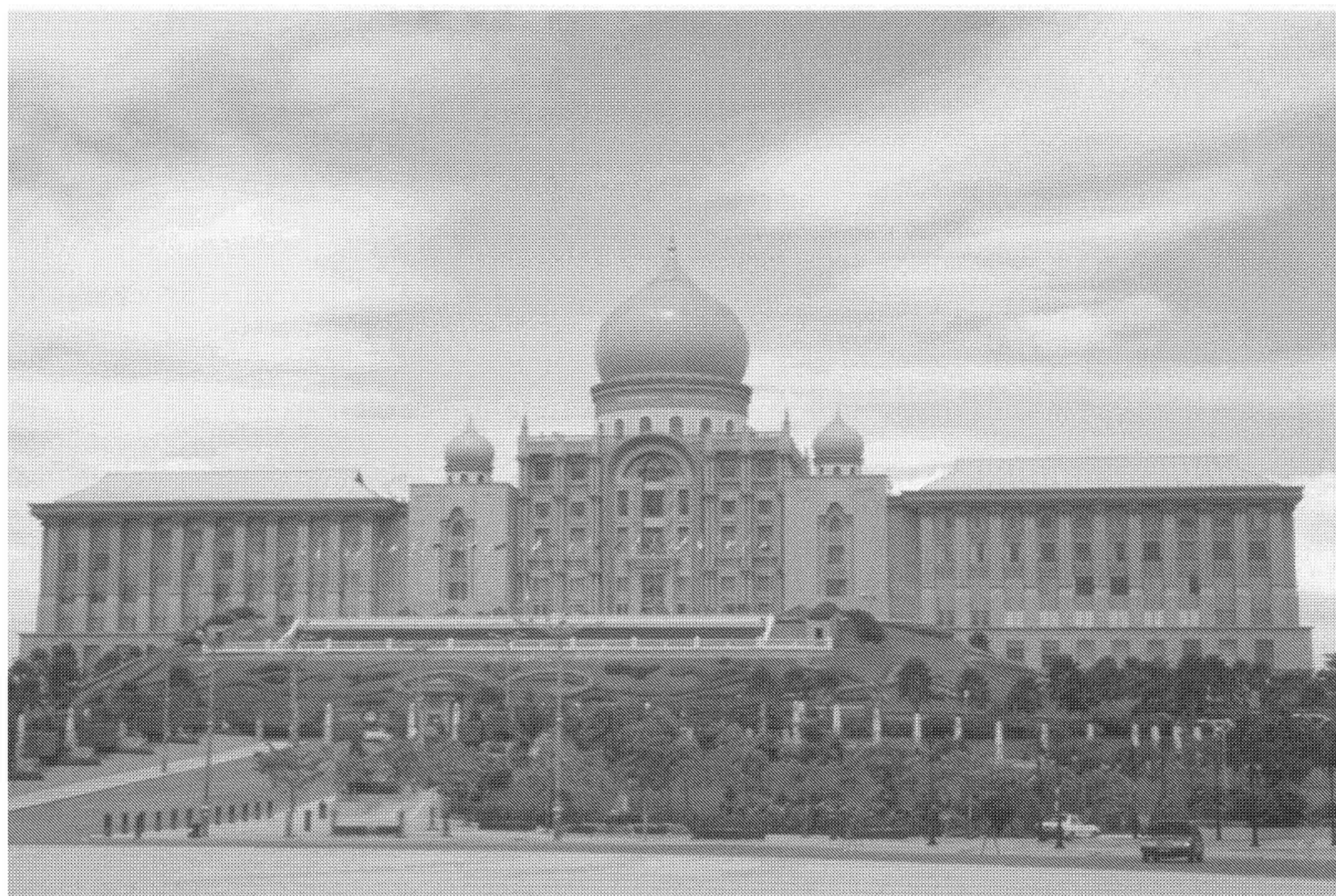
Fig. 28. Putrajaya. The new Parliament building for the Malaysian government.
