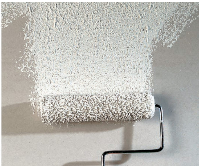
Texture paint applied with a roller.
