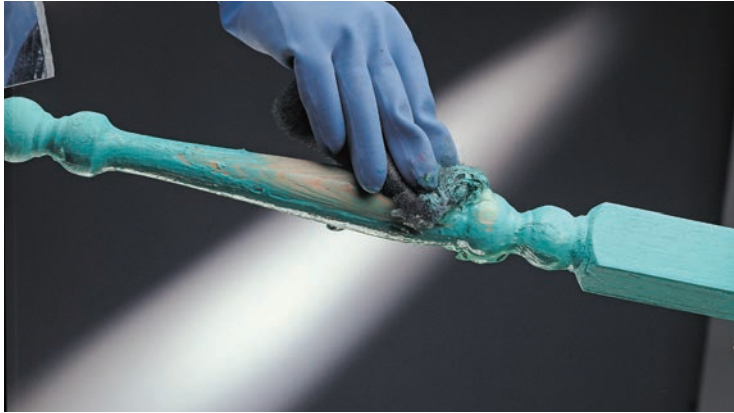
Solvent-based chemical stripper (in use).
