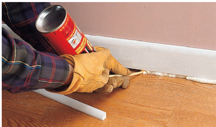
Spray foam insulation.
