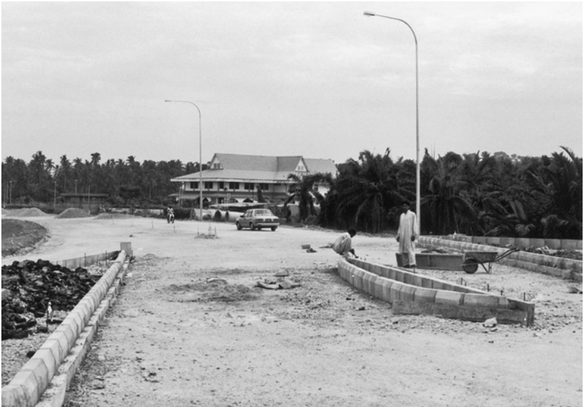
PLATE 16 New district office and road construction, Sugar Cane Village, 1997
