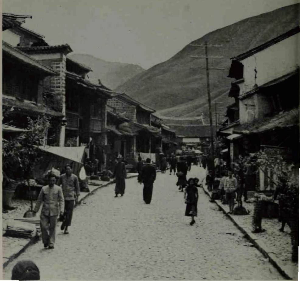
Street scene in Hsiakwan after repaving.
