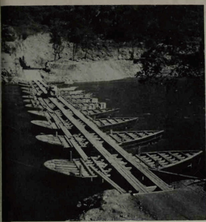
A pontoon bridge built on streamlined principle.
