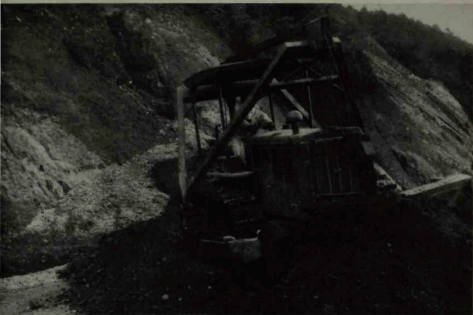
The clearing of a landslide with a bulldozer near Mangshih.
