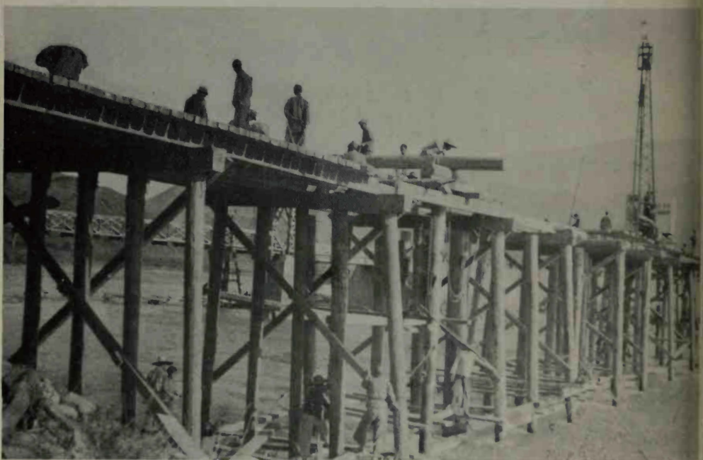
The building of the Yangpi Bridge with a Diesel pile-driver machine.
