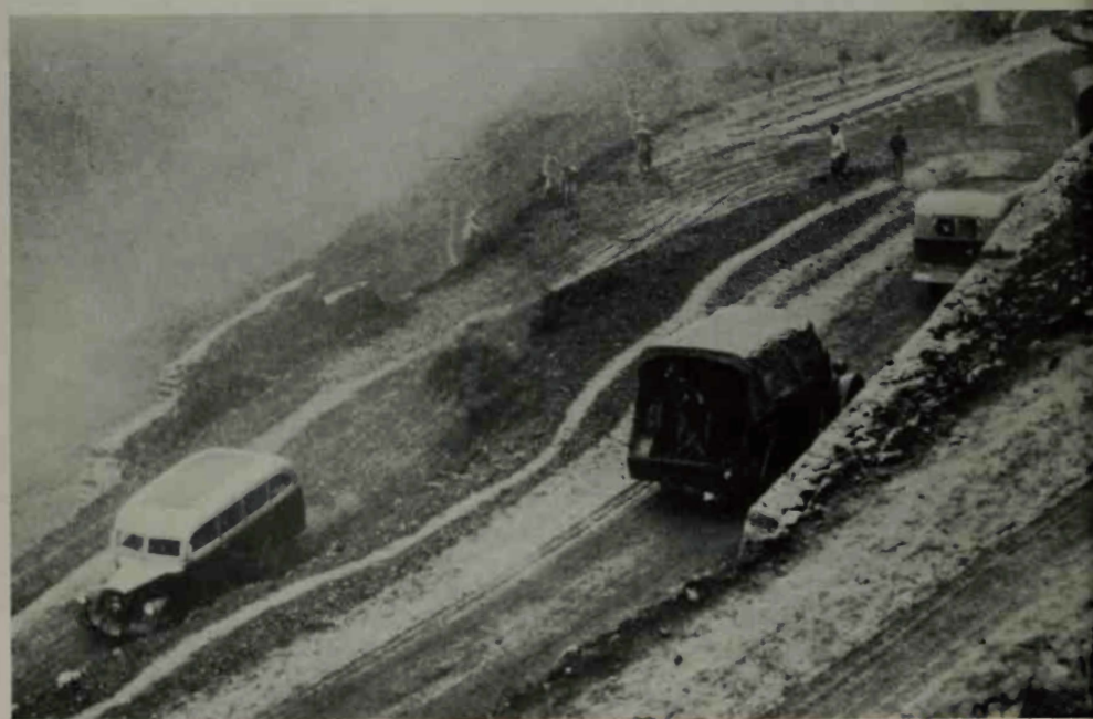
Many levels one above the other like this made the road vulnerable to landslides.
