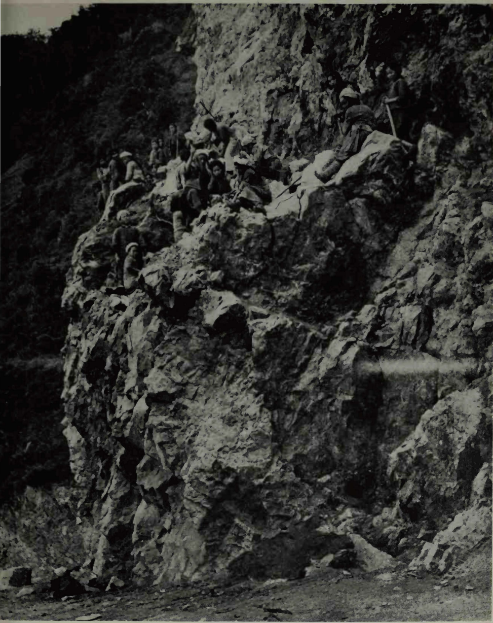
Workers cutting a way for the road through rock.
