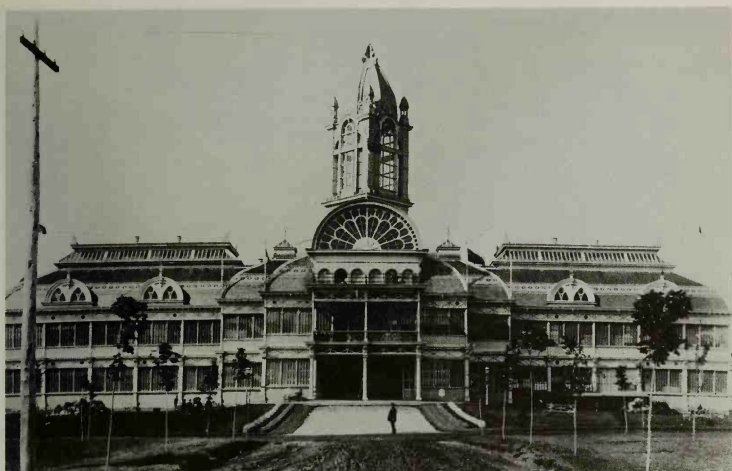
Above: Toronto's Second Crystal Palace (c. 1884) was actually a reconstruction of the first. The old structure of 1858 was disassembled in 1879 and carted to Exhibition Park, where a ground floor and an ungainly cupola plus other "busy" features were added. The total effect was the destruction of a strong, simple design and its replacement by a clumsy monstrosity.
