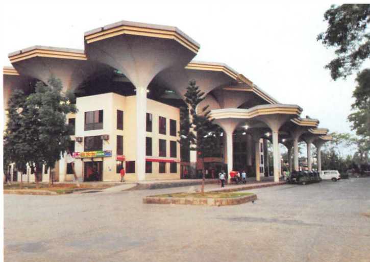
Sylhet Rail Station. Photo: Collection
