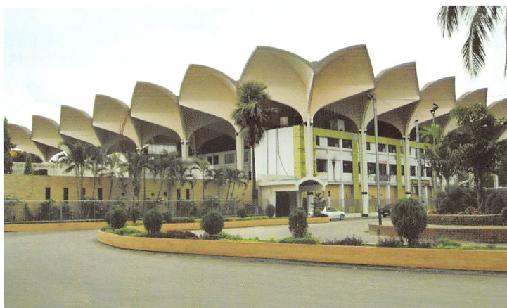
Kamalapur Railway Station. Photo. Collected
