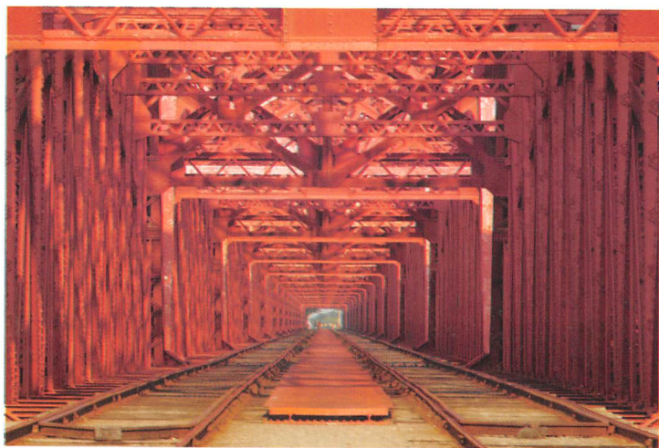
Hardinge Bridge over the mighty River Padma. Photo: Syed Zakir Hossain
