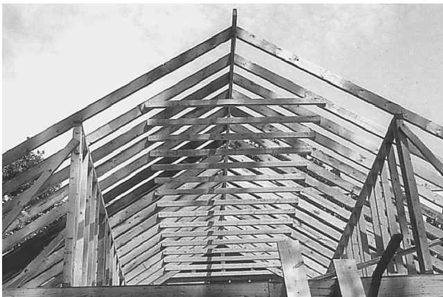
Fig. 1-50 Framing and supports for rafters.
