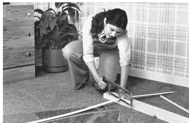
Fig. 13-50 Cutting the trim for the window. (Plaskolite.)
