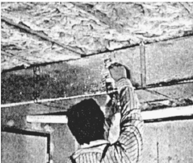
Fig. 6-50 Installing fiberglass on ductwork.
