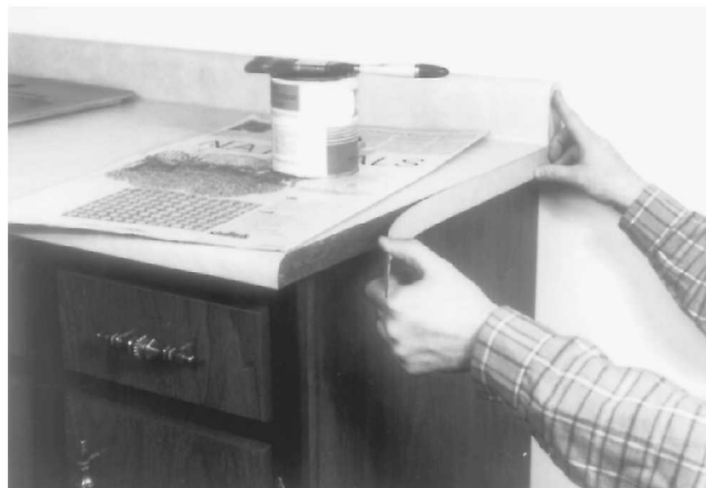
Fig. 15-47 Applying plastic laminate to countertops. I. Then cut out the opening. (Rockwell International Power Tool Division.) J. Mitered corners can be held with special clamps placed in cutouts on the bottom. (Formica.) K. Ends also may be covered by splashboards. (Formica.) L. Lay sink in opening. (Formica.) M. Ends may be covered by strips. (Formica.)
