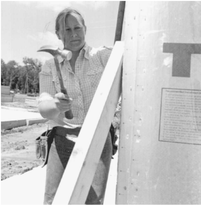
Fig. 6-39 Nailing a temporary brace.
