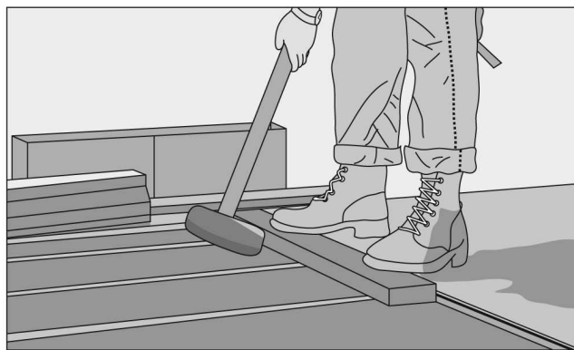
Fig. 5-51 A buffer board is used to protect the edges of tongue-and-groove panels.
