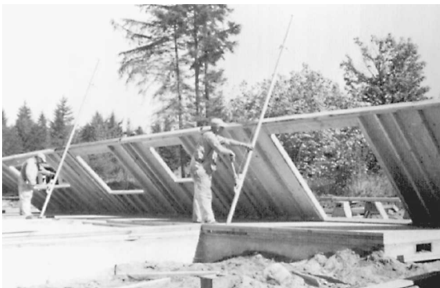
Fig. 6-35 Raising a wall section with wall jacks.
