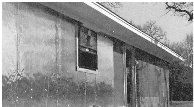
Fig. 6-56 Rigid polystyrene foam may be coated with reflective foil to increase its effectiveness as an insulation sheathing.
