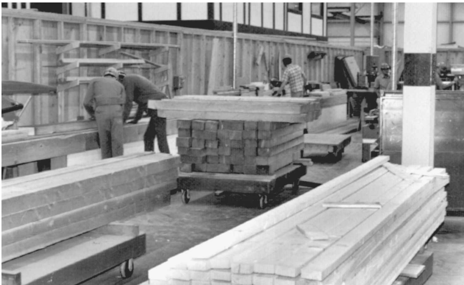
Fig. 18-14 Assembly line for pre-manufactured apartment house units. (Western Wood Products.)
