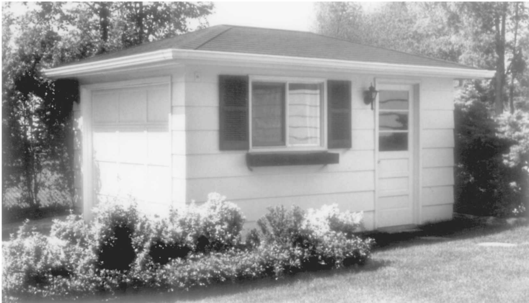
Fig. 17-105 View of one end of a storage shed.
