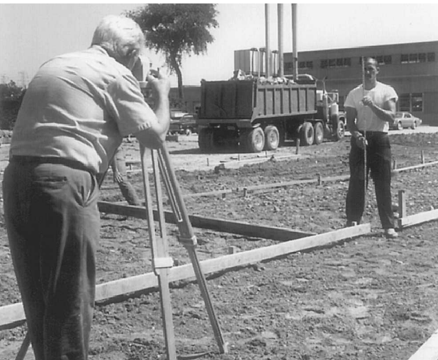
Fig. 4-20 Corners of forms are leveled before pouring the slab. (Portland Cement.)
