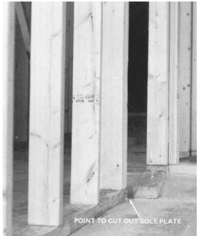
Fig. 6-44 At door openings, the partition soleplates are cut out after the wall is up.
