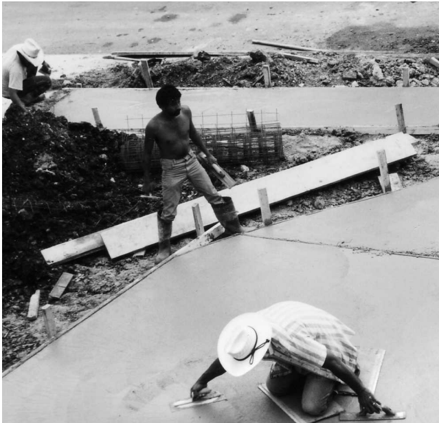
Fig. 4-25 Hand trowels may be used to smooth small surfaces.
