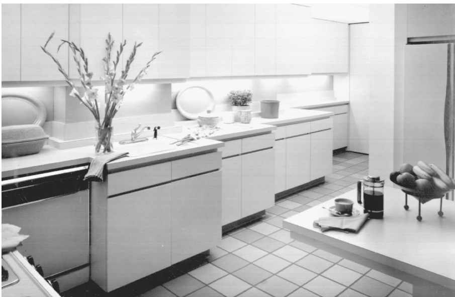
Fig. 15-26 Note the splashboards on these countertops.
