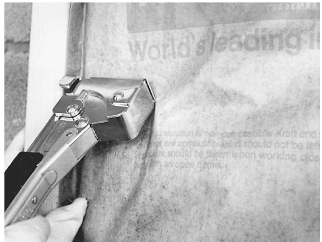
Fig. 13-30 Insert stapling. (Owens-Corning.)
