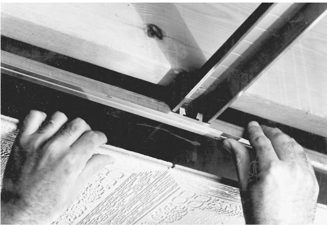
Fig. 14-54 Cross-T pieces then are attached to the runner to form a grid. (Armstrong Cork.)
