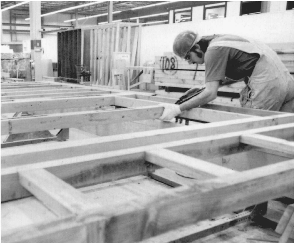
Fig. 18-16 Framing a wall panel. (Western Wood Products.)
