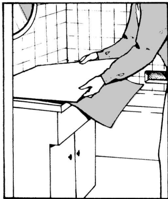
Fig. 17-34 Placing the glue-coated plastic laminate on the bottom over a piece of paper. (Grossman Lumber.)
