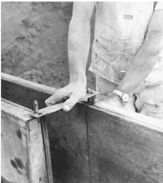
Fig. 3-28 Reusable forms are made from panels of plywood or metal. These special panel forms are assembled with special fasteners.
