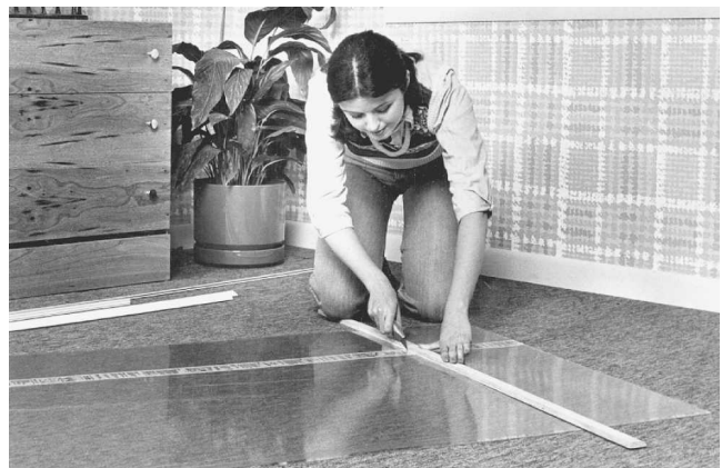
Fig. 13-49 Cutting the inside window. (Plaskolite.)
