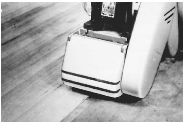
Fig. 15-75 After the floor is laid, it is sanded smooth using a special sanding machine. (National Oak Flooring Manufacturers Association.)
