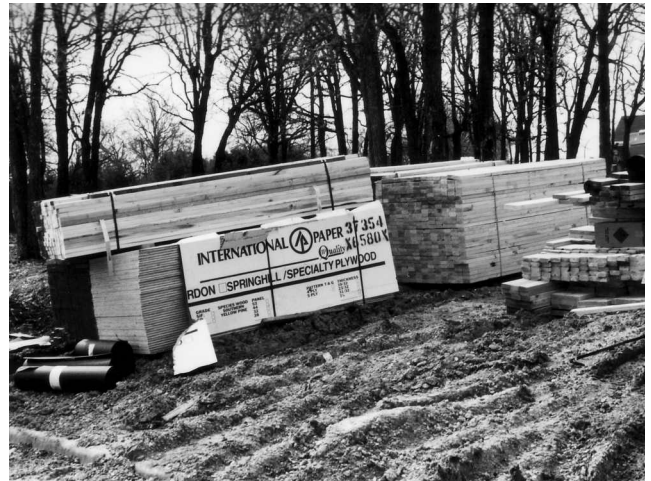
Fig. 2-33 B. Bundled lumber delivered to the building site.
