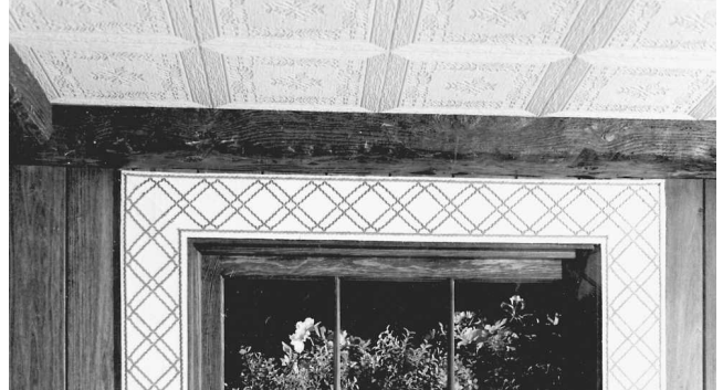
Fig. 14-57 No metal grid shows when grooved-edge tile is used. (Armstrong Cork.)
