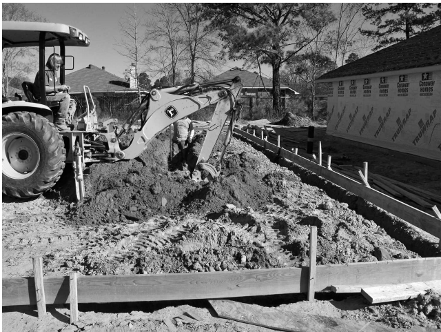
Fig. 4-5 Forms are erected.
