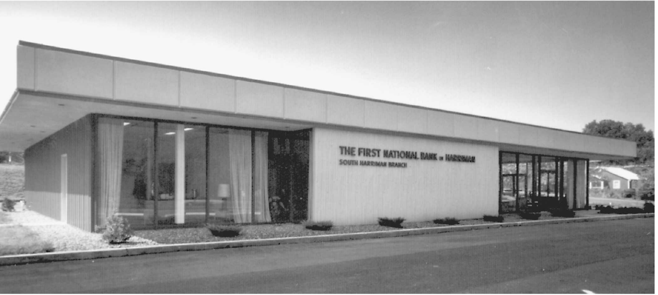
Fig. 18-13 Commercial building made in a factory and assembled on site. (Butler.)
