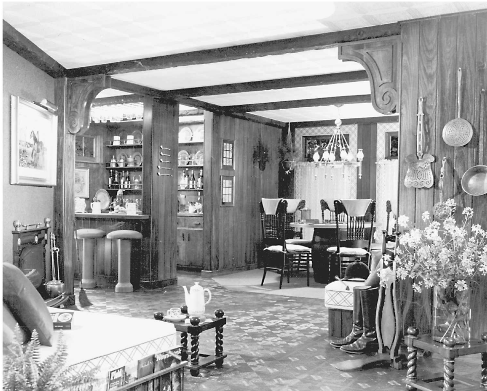
Fig. 14-50 A basement area using ceiling tile and artificial beams and posts. (Armstrong Cork.)
