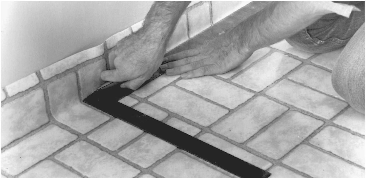
Fig. 17-43 Use a utility knife and carpenter's square to make sure that the cut is straight. (Armstrong Cork.)
