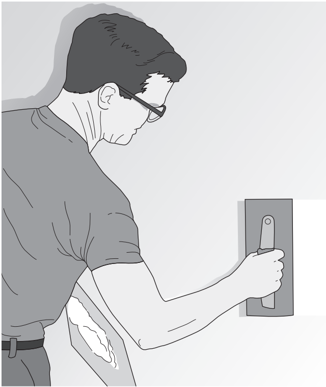
Fig. 14-47 Plaster being applied with a trowel. (Gold Bond.)
