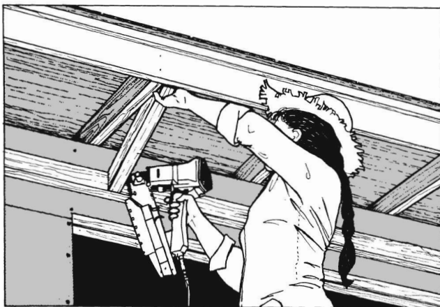
Fig. 7-2 Braces (lookouts) are put in where they are needed. (Duo-Fast.)
