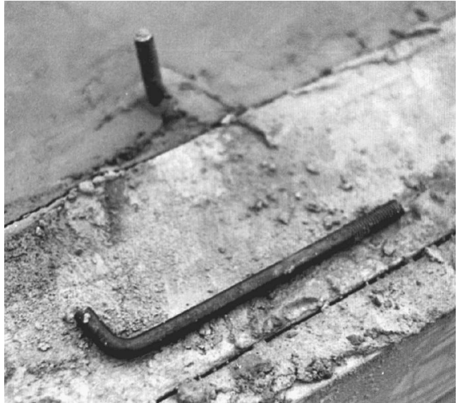
Fig. 4-27 Anchor bolts are embedded into the foundation wall.
