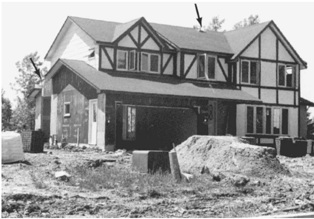
Fig. 7-88 Arrows show the openings in the roof for the chimney.
