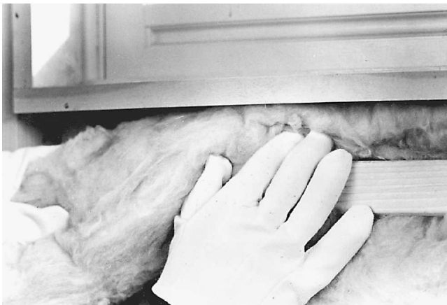
Fig. 13-33 Filling small gaps. (Owens-Corning.)
