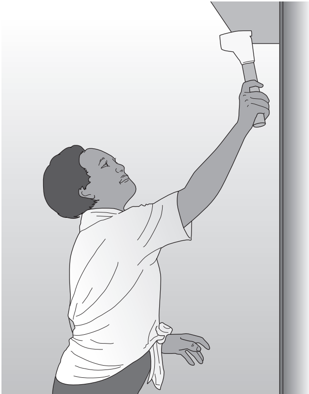
Fig. 10-55 Panel siding is often stapled in place.
