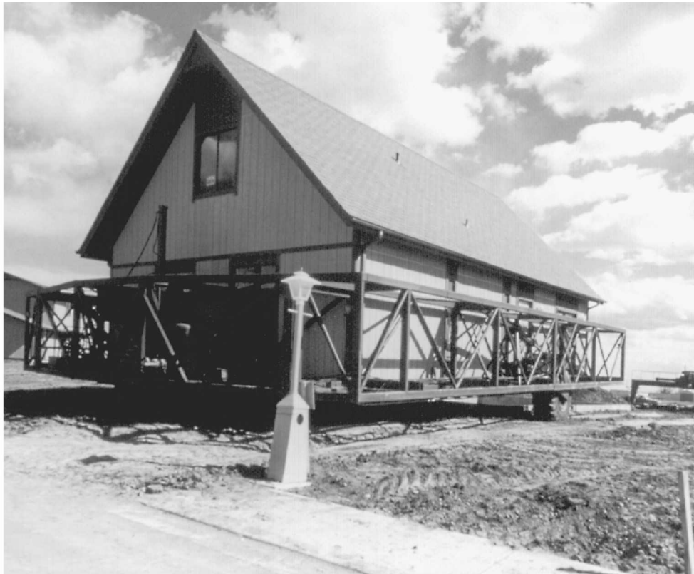
Fig. 18-23 A machine moves the house over the foundation. (Western Wood Products.)
