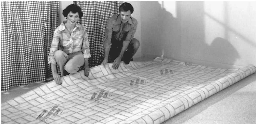
Fig. 17-42 Unroll the flooring and allow it to sit face up overnight before installing it. (Armstrong Cork.)
