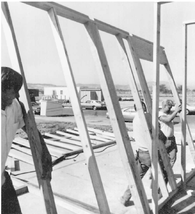
Fig. 6-34 Raising a wall section by hand.
