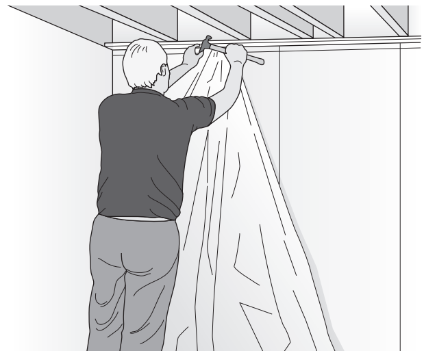
Fig. 14-34 A vapor barrier is applied over a concrete wall. This is a must for best paneling. (Masonite.)
