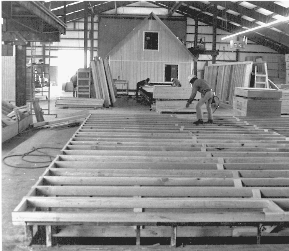
Fig. 18-20 Floor joists being laid for a manufactured house. (Western Wood Products.)
