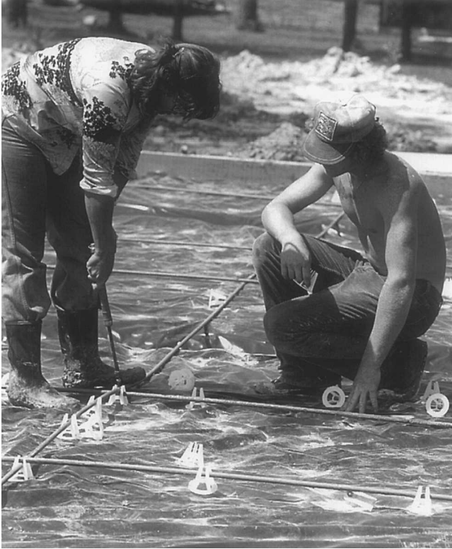
Fig. 4-16 Chairs hold rebar in place for pouring.
