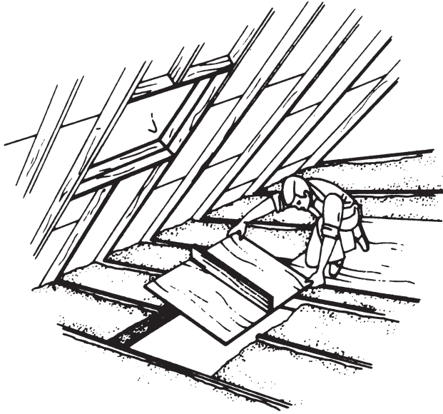
Fig. 9-64 Removing the ceiling section. (Novi.)
