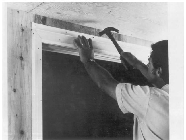
Fig. 9-139 Exterior nailing of the unit. (Andersen.)
