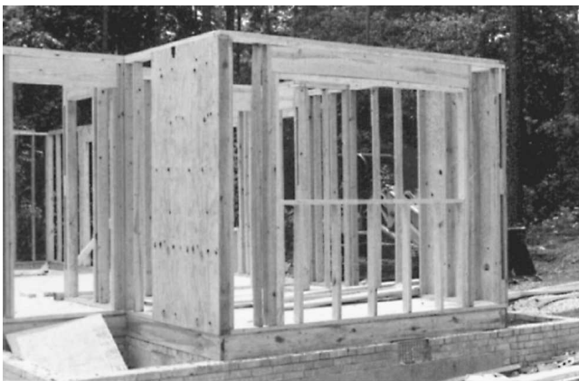
Fig. 6-1 Wall frames are put up after the floor is built.
