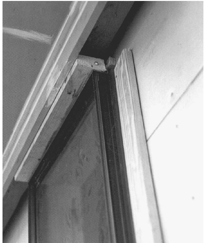
Fig. 10-3 A window unit blocked for brick siding.
