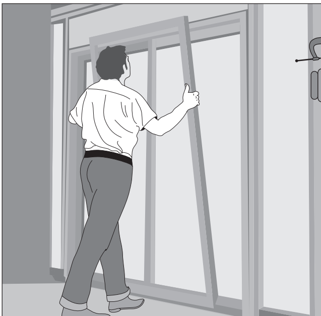
Fig. 9-146 Placing the operating door on the rib of the metal sill facing. (Andersen.)
