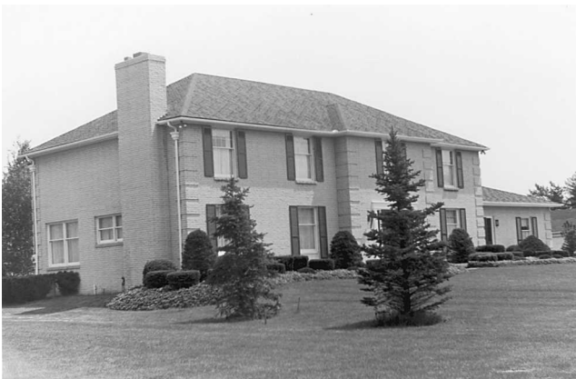
Fig. 8-3 Hip-and-valley roof.
