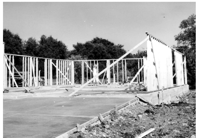
Fig. 6-38 Once raised, walls are held in place with temporary braces.
