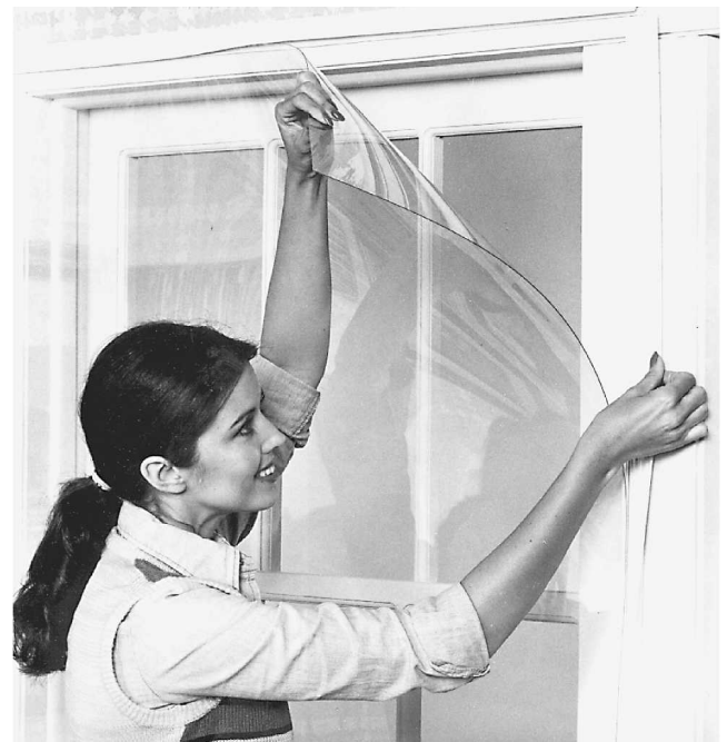
Fig. 13-54 Placing the plastic inside the window.
