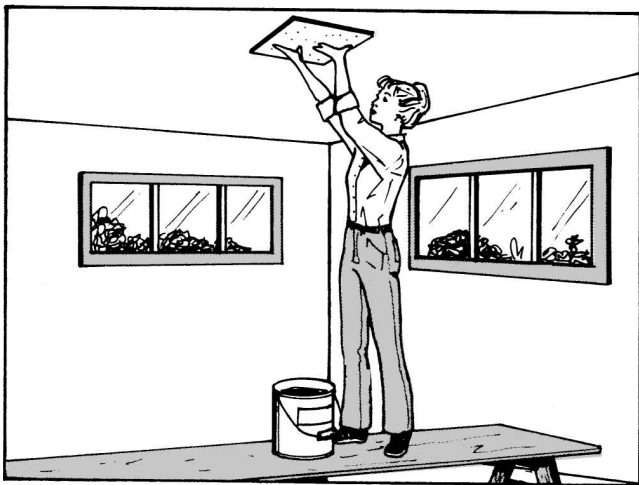
Fig. 17-60 Apply the first tile where the lines cross on the ceiling. Work toward the edges. (Grossman Lumber.)
