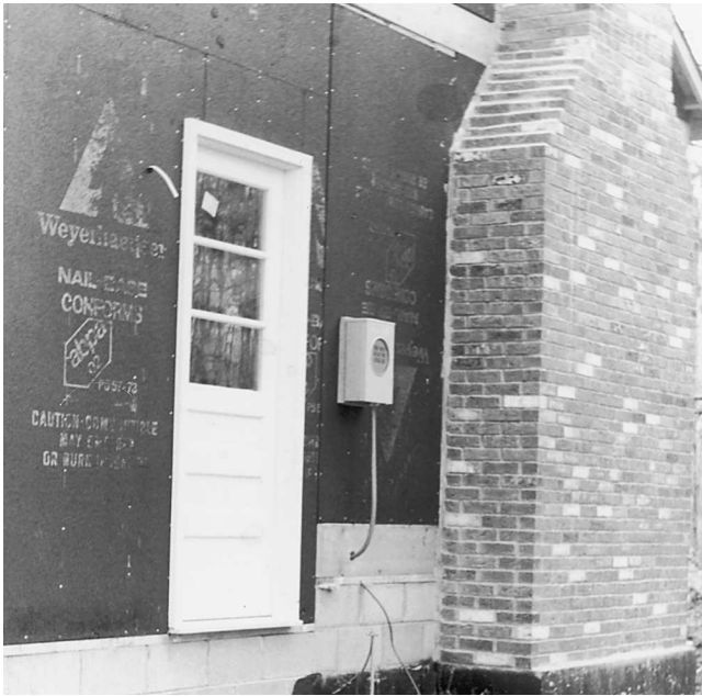
Fig. 9-76 A prehung exterior door with three panels of glass. Note how the trim sticks out sufficiently for the siding to butt against it.
