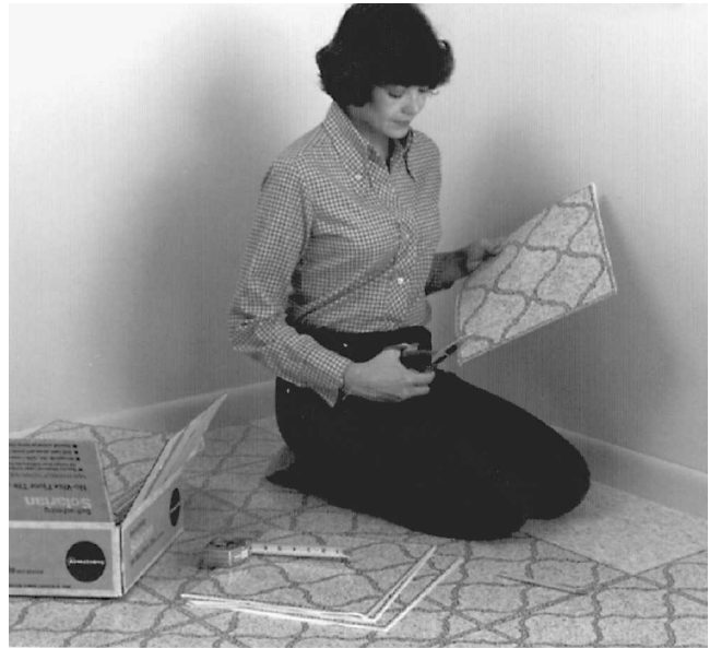
Fig. 17-49 Border tiles for the edges of the room can be easily cut to size with a pair of household shears. (Armstrong Cork.)
