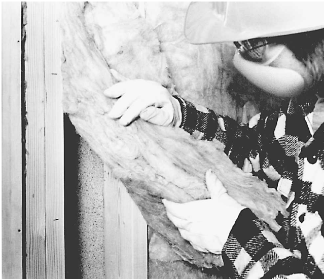
Fig. 13-36 Filling narrow stud spaces. (Owens-Corning.)
