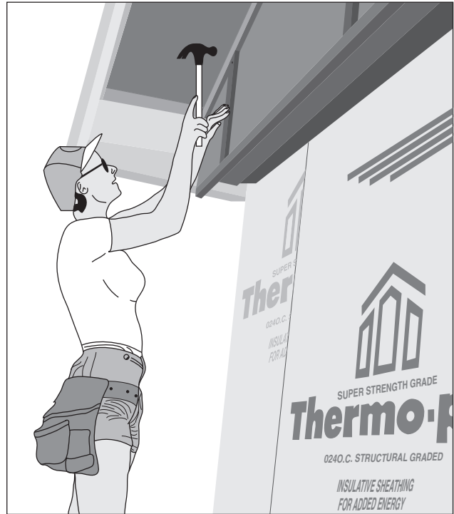
Fig. 10-38 Gable siding is done before wall siding.
