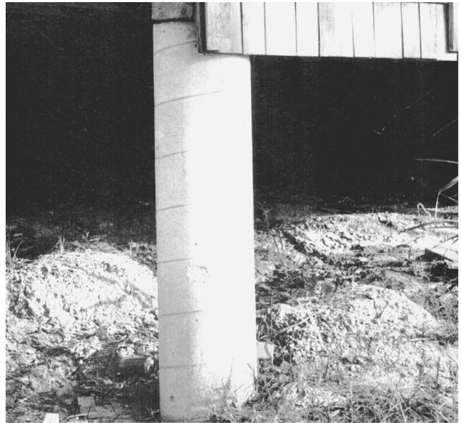
Fig. 3-32 A round form made of cardboard.
