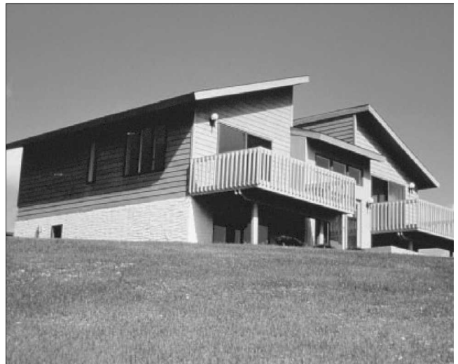
Fig. 22-28 The PWF exterior foundation walls blend with the rest of the house.
