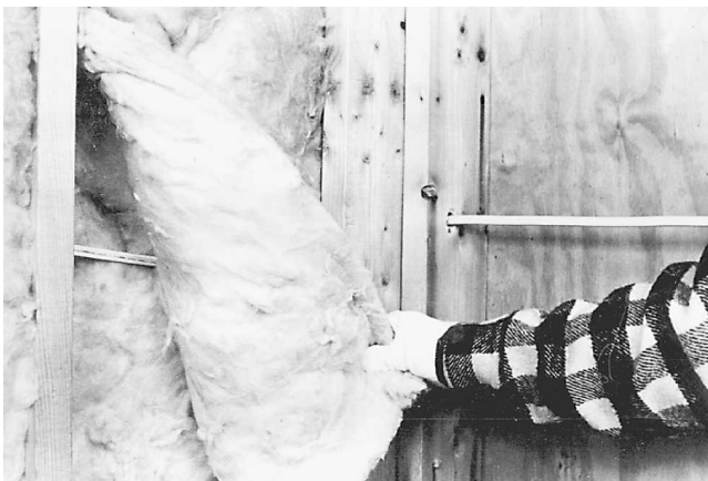
Fig. 13-37 Insulation around wiring. (Owens-Corning.)
