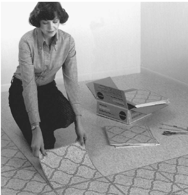
Fig. 17-48 Do one section of the room at a time. The tiles can be maneuvered into position and pressed into place. (Armstrong Cork.)
