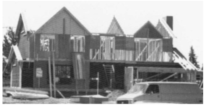
Fig. 7-95 Erection of sidewalls to a house.
