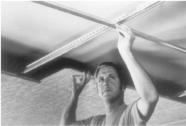
Fig. 17-68 Continue across the room in this manner. Insert the tiles and cross T's. (Armstrong Cork.)
