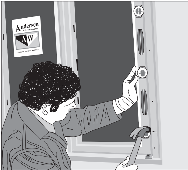
Fig. 9-42 Check for plumb, and nail the lower corner.
