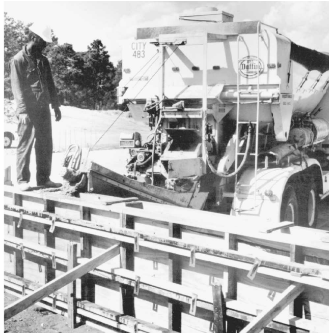
Fig. 3-39 Concrete is poured or pumped into the finished form.
