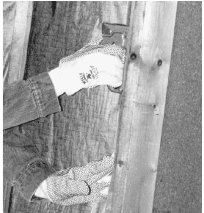
Fig. 14-3 Insulation is stapled between the studs.
