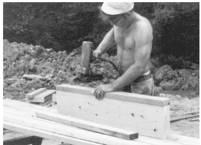
Fig. 6-23 Nailers can be used to assemble headers.
