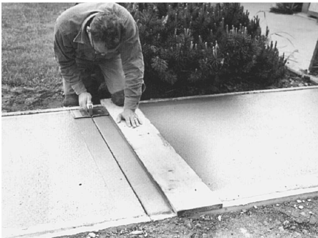
Fig. 4-29 Joints may be troweled into a surface.
