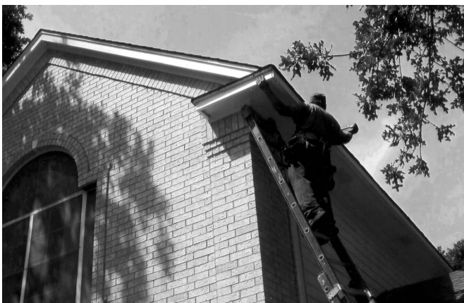
Fig. 17-41 A. How to select the right fittings and the right quantity. (Sears, Roebuck and Co.) B. Extruding the one-piece gutter from a roll of aluminum located inside the truck. C. Shorter pieces ready for mounting on the fascia board. D. Mounting the gutter using one person to do the job.
