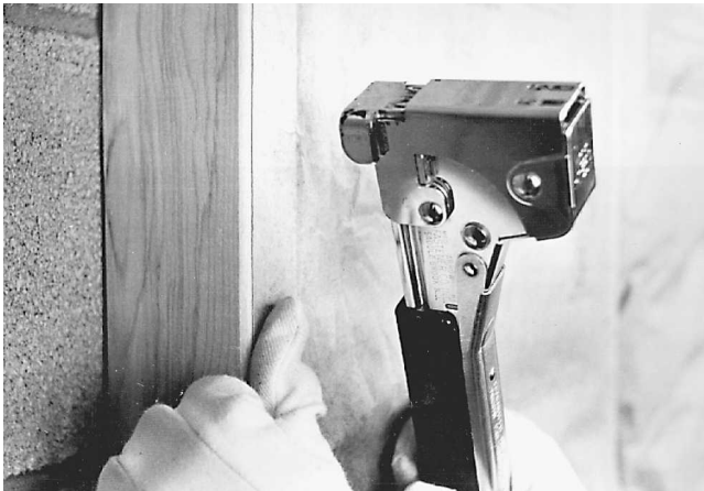
Fig. 13-31 Faced stapling. (Owens-Corning.)
