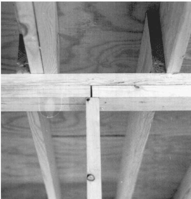
Fig. 6-5 Top plates are spliced over a stud.
