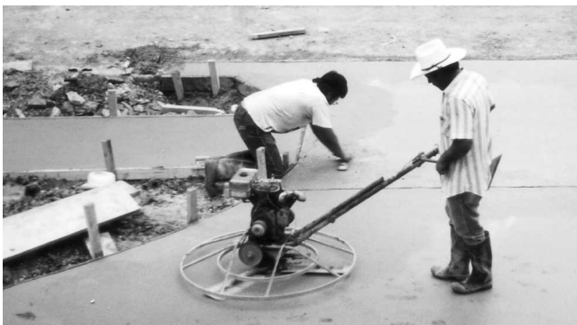
Fig. 4-26 A power trowel is used to finish large surfaces.
