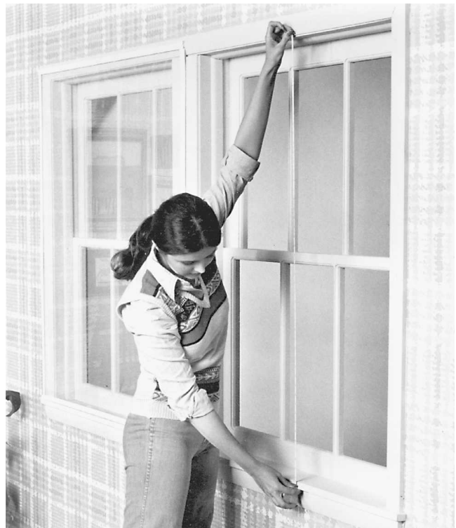
Fig. 13-48 Measuring for the inside storm window. (Plaskolite.)
