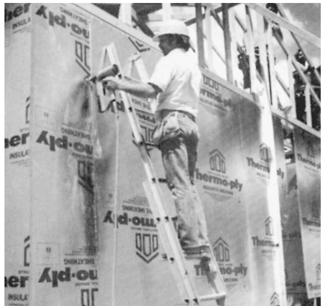
Fig. 6-57 Another type of energy-efficient sheathing is similar to rigid foam but is coated with reflective foil. (Simplex.)
