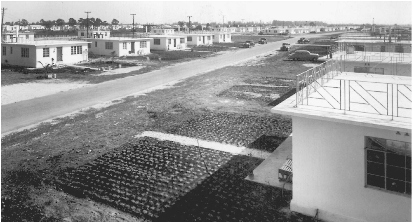
Fig. 18-11 Poured concrete houses. Example of an early type of manufactured house. (Universal Form Clamp.)
