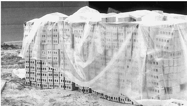
Fig. 2-36 Storing bricks on site.
