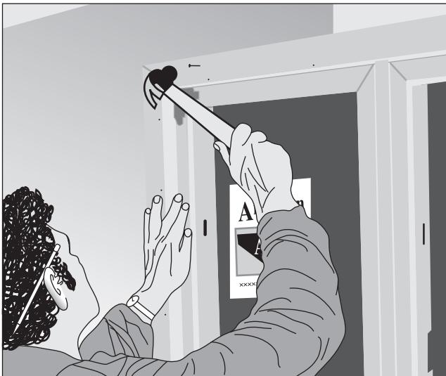
Fig. 9-40 Use 3½-inch nails to partially secure one corner through the head casing. (Andersen.)
