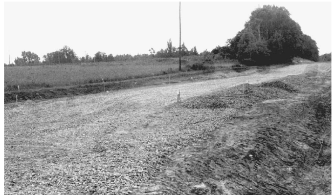
Fig. 1-42 The beginning of a street.
