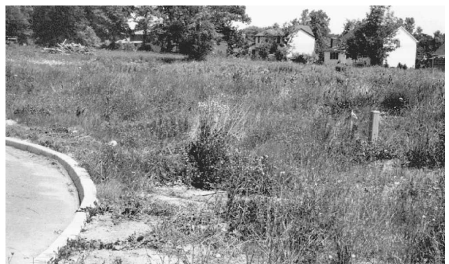
Fig. 1-43 Locating a building site and removing the curb for the driveway.
