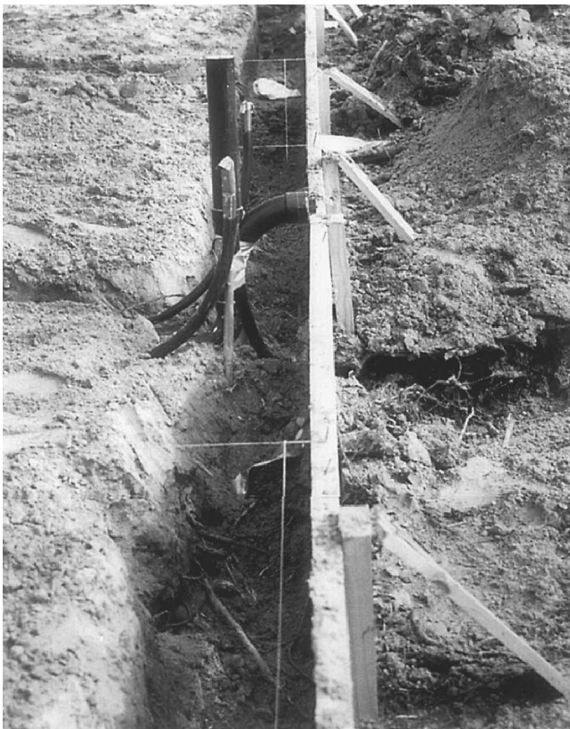
Fig. 4-11 Sand is leveled. Use chalk lines as guides.
