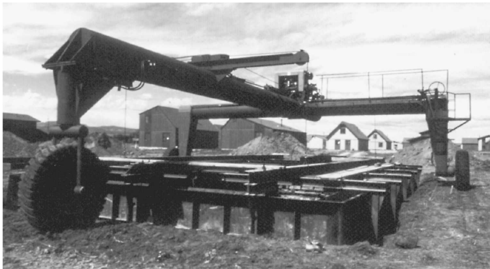
Fig. 18-22 A machine laying the foundation. (Western Wood Products.)
