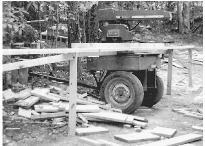
Fig. 6-18 A radial arm saw can be used on the site.
