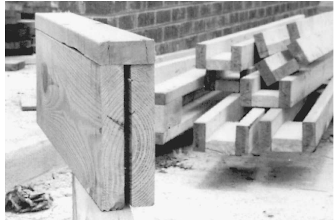
Fig. 6-22 Use 1/2-inch plywood for spaces between headers.
