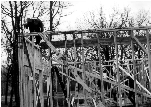
Fig. 6-28 Nailing studs for wall frames.
