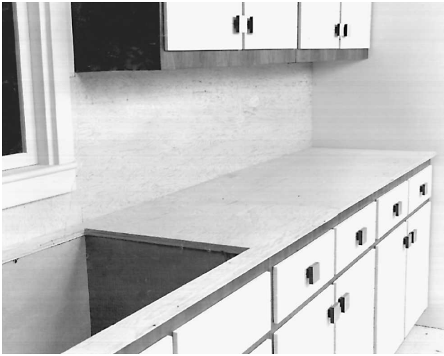
Fig. 15-24 Plywood base installed for the application of countertop tile. (American Olean Tile.)
