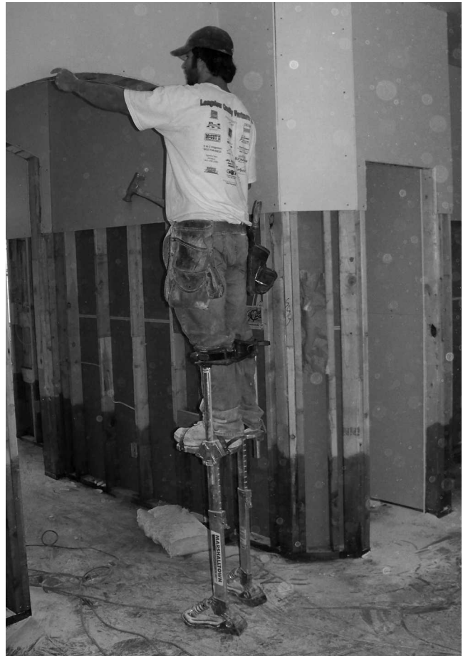
Fig. 14-28 Taping and bedding Sheetrock seams.
