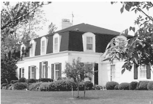
Fig. 8-68 Mansard roof.
