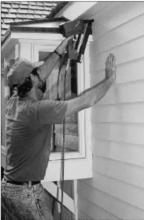
Fig. 22-27 Application of siding.
