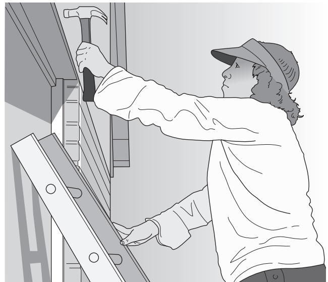
Fig. 10-39 Installing gable siding.
