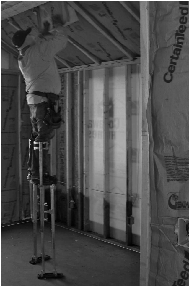
Fig. 14-13 Stilts are often used for nailing and finishing ceilings. (Goldblatt Tools.)
