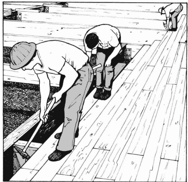
Fig. 16-71 Widely spaced floor or roof joists are decked with long planks. (Weyerhaeuser.)
