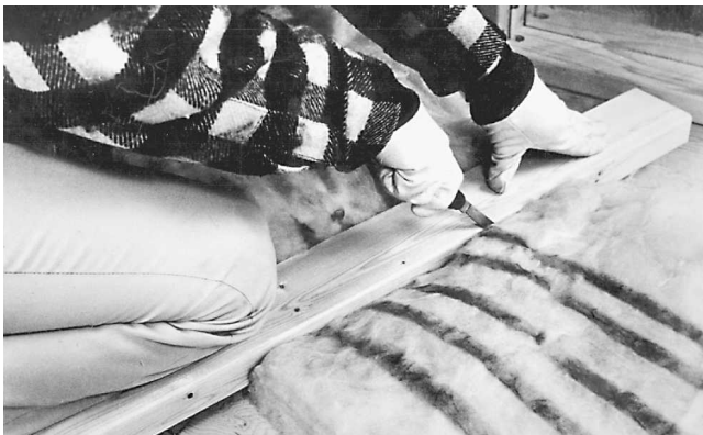
Fig. 13-28 Cutting Fiberglas insulation. (Owens-Corning.)
