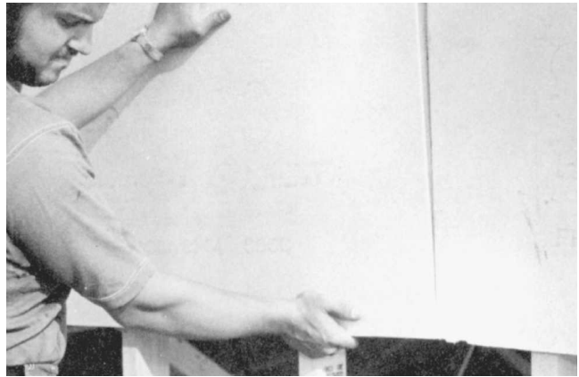
Fig. 6-55 Rigid polystyrene foam sheathing provides more insulation. (Dow Chemical.)
