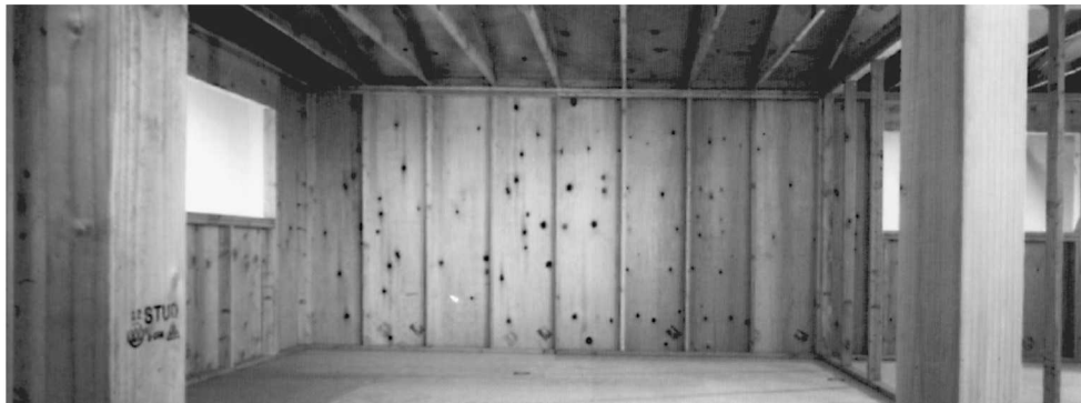
Fig. 18-1 Building materials used in construction are changing. Note the extensive use of plywood in a modern house. (Western Wood Products.)
