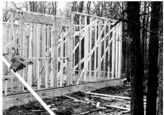
Fig. 6-37 Wall sections are anchored to slabs after being erected.
