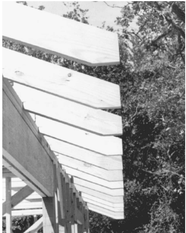
Fig. 1-23 Rafter overhang cut to a given angle.
