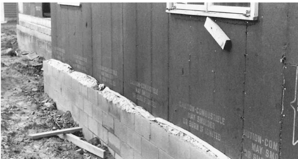
Fig. 18-2 Carpenters must learn to adapt to new materials like this composition nail base used for siding.
