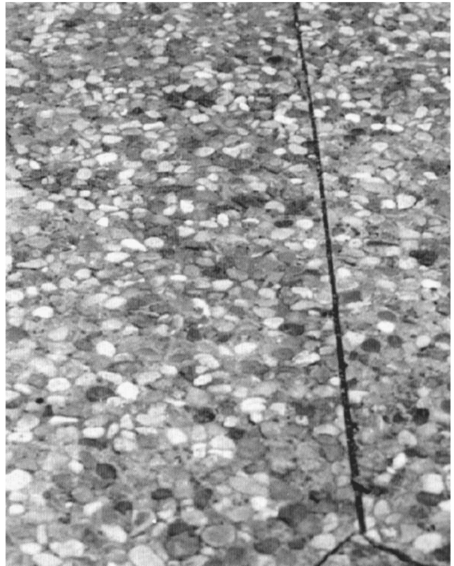
Fig. 4-30 Some joints may be cut with saws.
