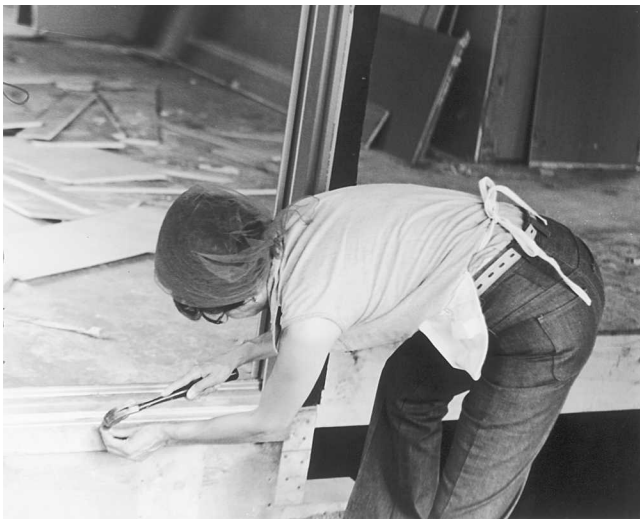
Fig. 9-141 Applying the sill support under the metal sill facing.
