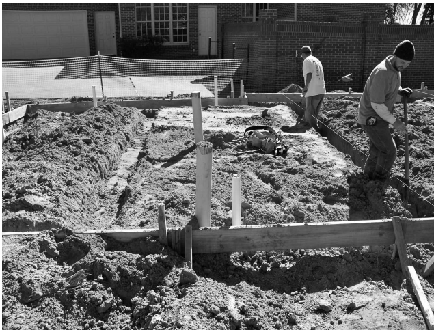
Fig. 4-9 Excavations are also made for footings in the slab.
