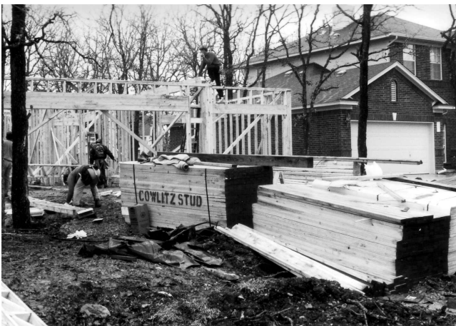
Fig. 6-15 Precut studs ready at a site.
