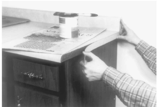
Fig. 17-35 Applying plastic laminate to countertops. I. Then cut out opening. (Rockwell International Power Tool Division.) J. Mitered corners can be held with special clamps placed in cutouts on the bottom. K. Ends also may be covered by splashboards. L. Lay sink in opening. M. Ends may be covered by strips. (Formica.)
