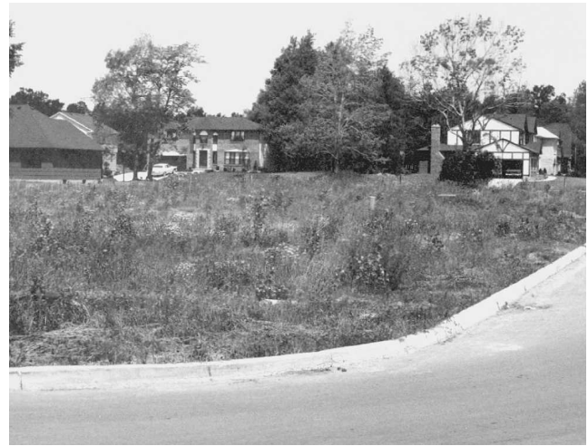
Fig. 2-3 Rough-cleared lot. Only weeds need to be taken out as the basement is dug.
