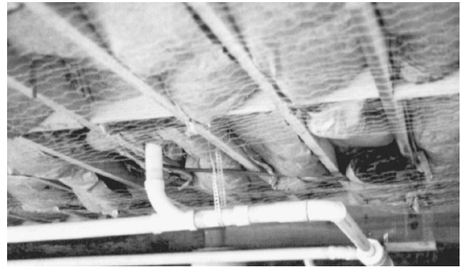
Fig. 5-63 Insulation between floor joists should be supported.
