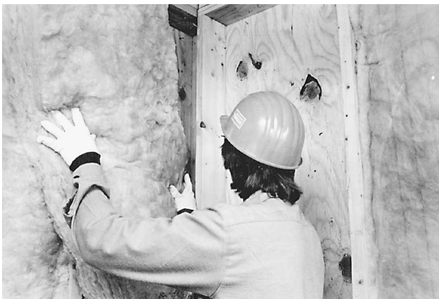
Fig. 13-32 Installing unfaced insulation. (Owens-Corning.)
