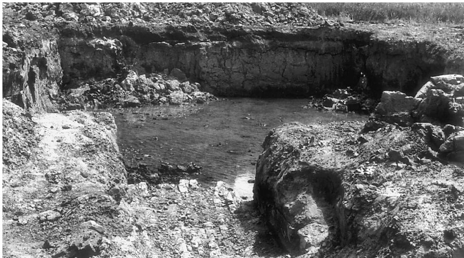
Fig. 2-32 Excavation for a basement.
