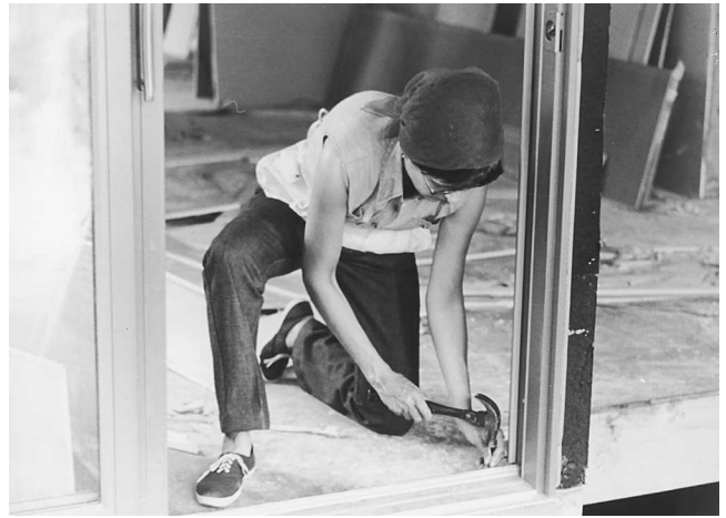
Fig. 9-138 Securing the sill to the floor by nailing.
