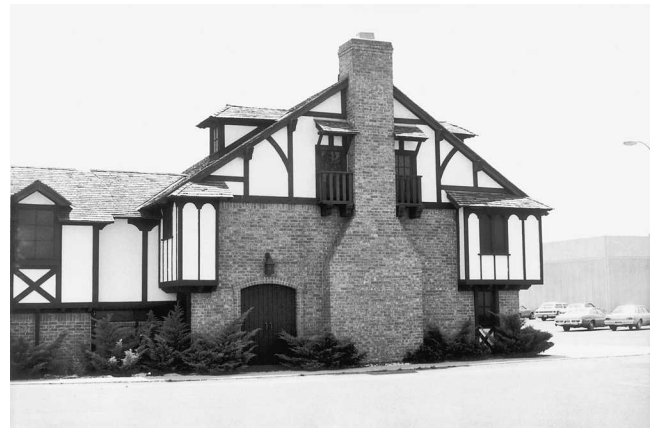
Fig. 10-35 Smooth gable panels contrast with the brick siding.
