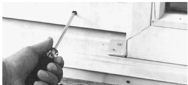
Fig. 9-148 Adjusting the door for square. (Andersen.)
