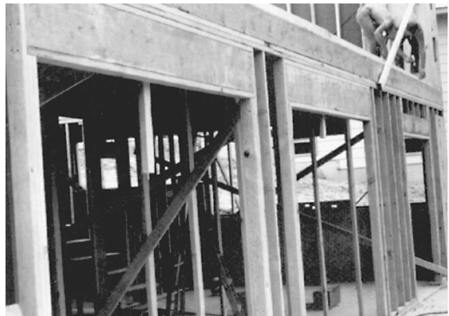
Fig. 6-16 Solid headers may be used instead of cripples.
