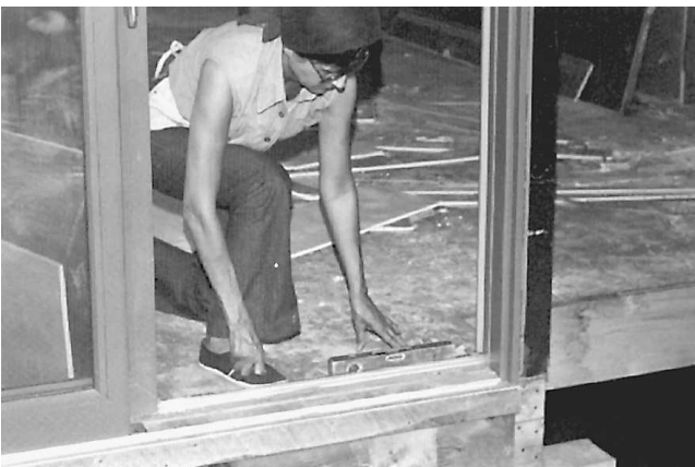
Fig. 9-137 Leveling the sill.
