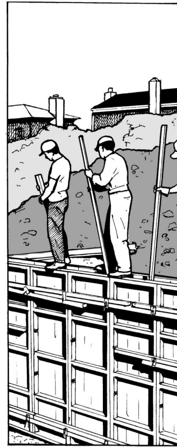
Fig. 3-23 Concrete is tamped into forms to get rid of air pockets. (Portland Cement.)
