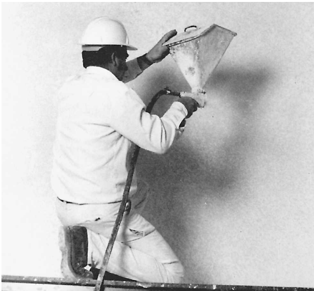
Fig. 14-48 Plaster being applied by machine. (Gypsum Association.)
