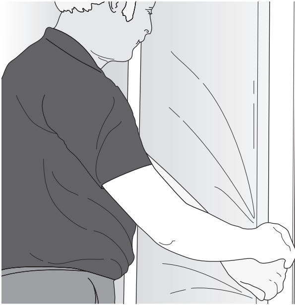
Fig. 14-36 Insulation is added between the furring strips.
