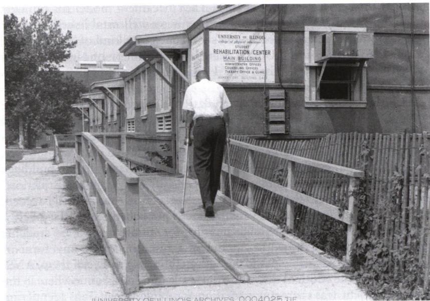
FIGURE 3.1 Ramped entrance at the first Rehabilitation Center on the campus of the University of Illinois. In spite of its wheelchair-accessible entry, the building was marked by minimal signage, c. 1956. Courtesy University of Illinois.
