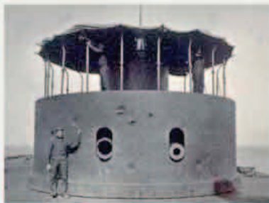
DAMAGED MONITOR TURRET
