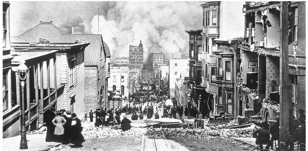
Crumbling buildings lined the streets after the earthquake.
