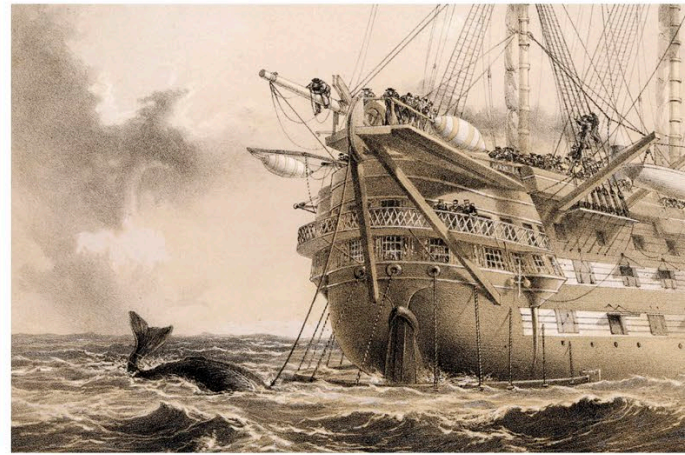
Laying cables under the Atlantic Ocean
