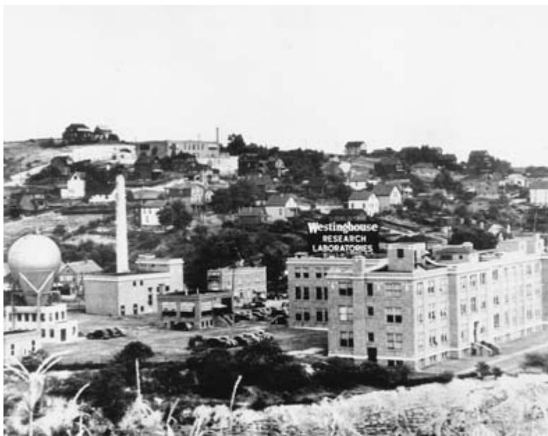
FIGURE 4. The Westinghouse Research Laboratories in Forest Hills, Pennsylvania, ca. 1937. The facility had been built in 1916, several miles distant from the company's East Pittsburgh production plant. To the left is the company's "atom smasher," a Van de Graaff-type accelerator, which had just been constructed and which signified leadership in industrial nuclear physics. The physicist E. U. Condon had been hired as associate director of the laboratory, given broad authority to build up a large-scale program in fundamental research. (Reproduced by permission of the American Institute of Physics, Emilio Segrè Visual Archives and Westinghouse.)
