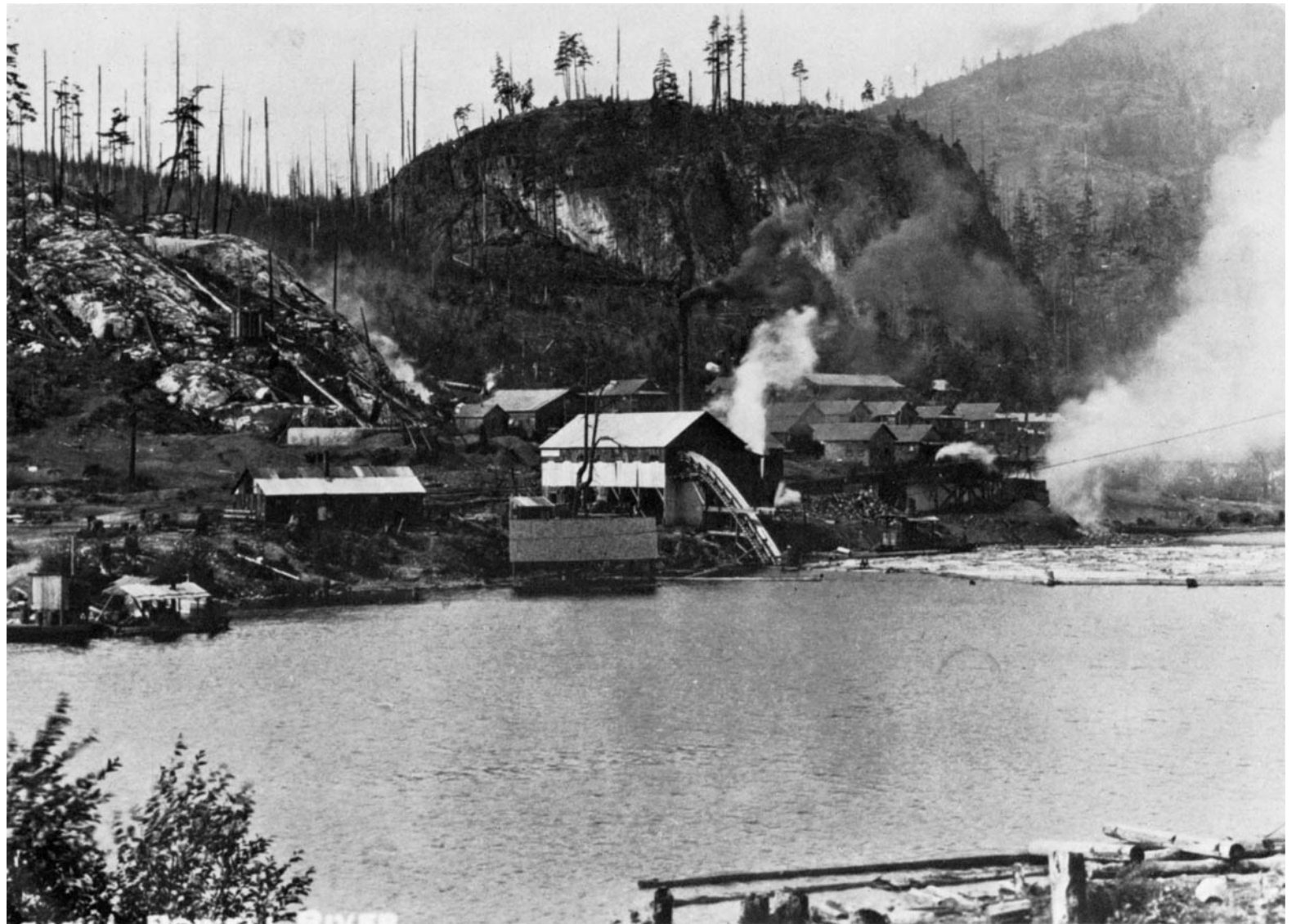
The first Powell River mill under construction, 1911.
