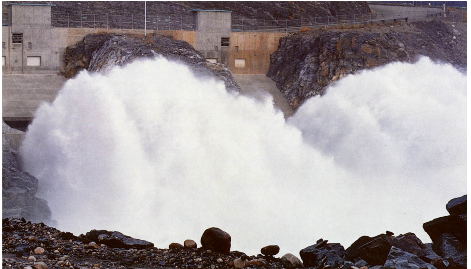
This tailrace at Mica dam indicates the hydraulic force that generates hydroelectric power.
