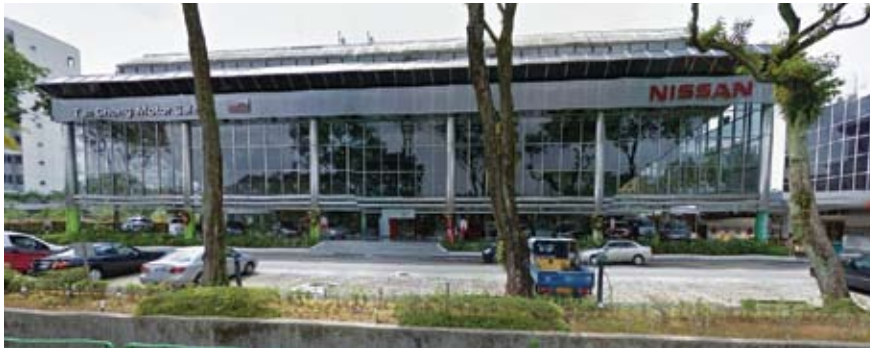
Lee Soon on his design for the Tan Chong Motors showroom on Bukit Timah Road: "I deliberately made it slightly slanted so that the cars in the showroom did not reflect off the cars passing by thus blinding motorists."
