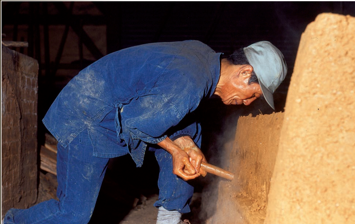
The murage pushes a long pole through the wall to create observation ports.
