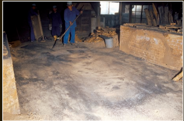
After firewood is burned, the ground and burned wood are pounded with wooden poles for about 40 minutes to produce a dry, flat surface that becomes the foundation of the furnace. When the tataru is running, the floor reaches very high temperatures, and steam will be visible.
