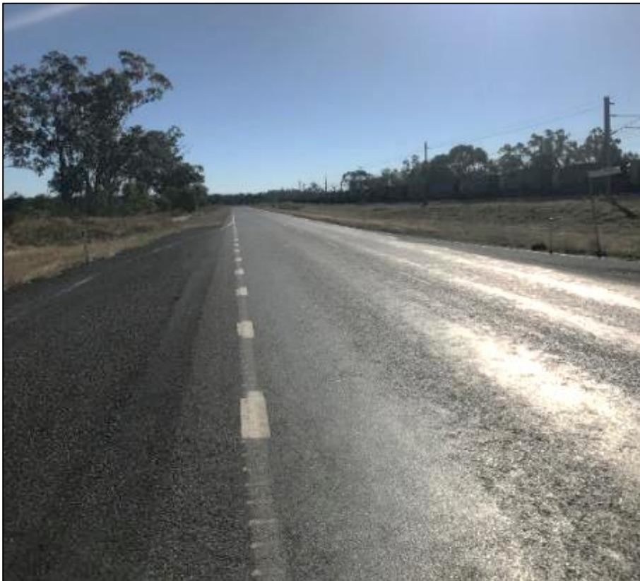
Source: Site Investigation conducted by Cardno on 16 th July 2019
