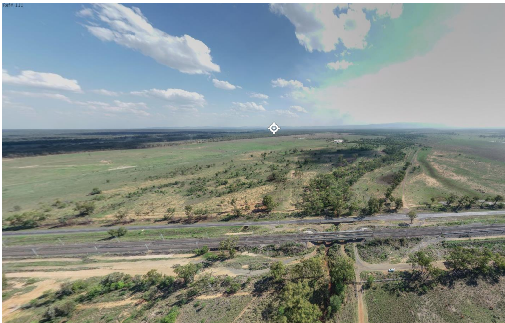
Figure 4.6 - Drone photograph looking south across along Charlevue Creek across the Capricorn Highway to the Project area (source: Magnetic South Pty Ltd)
