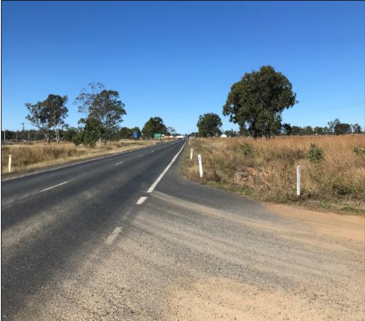
Source: Site Investigation conducted by Cardno on 16 th July 2019
