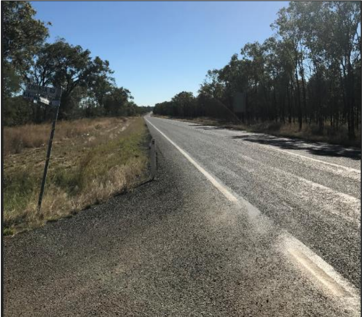
Figure 3-3 Capricorn Highway / Cooinda Road Intersection
