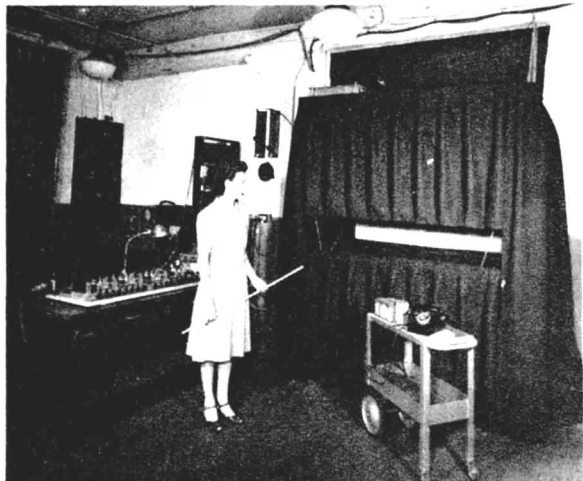
On the table at left is the system of filters and amplifiers; the long-persistence fluorescent belt is visible between curtains.
