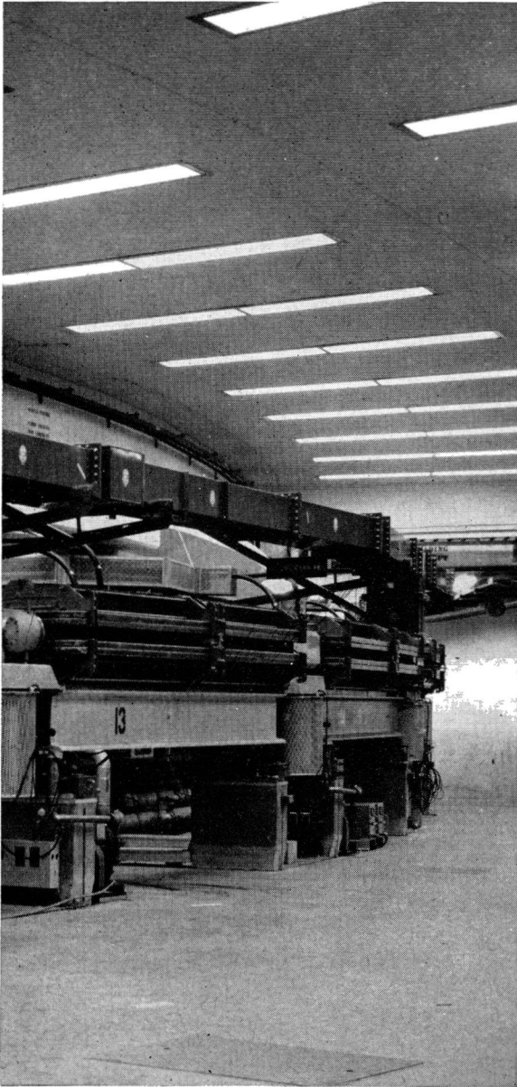
Fig 6. A segment of the ring, 236 feet in diameter, in the shielding tunnel, March, 1962. The electrons orbit in a stainless steel track that runs between the jaws of 48 C-shaped electromagnets. Several sections appear in this shot; each magnet is twelve feet long, set on the numbered steel beams resting on the reinforced concrete pillars. (The reinforcing rods for these pillars appear protruding from the floor in Fig. 5) At the extreme left is one of the sixteen radiofrequency resonant cavities which applies the accelerating potentials to the electrons; each one gives two kicks to the electrons on each pass—and the electrons make 10,000 passes!—as they move from end to end of the cavity. (Remember the electrons are moving at a speed so close to c , the velocity of light, as to be practically indistinguishable from it.) The cavities are resonant at 475 megacycles; they're fed by the big rectangular wave guides from high-power klystrons banked at the powerhouse in the center of the tunnel's circle.
