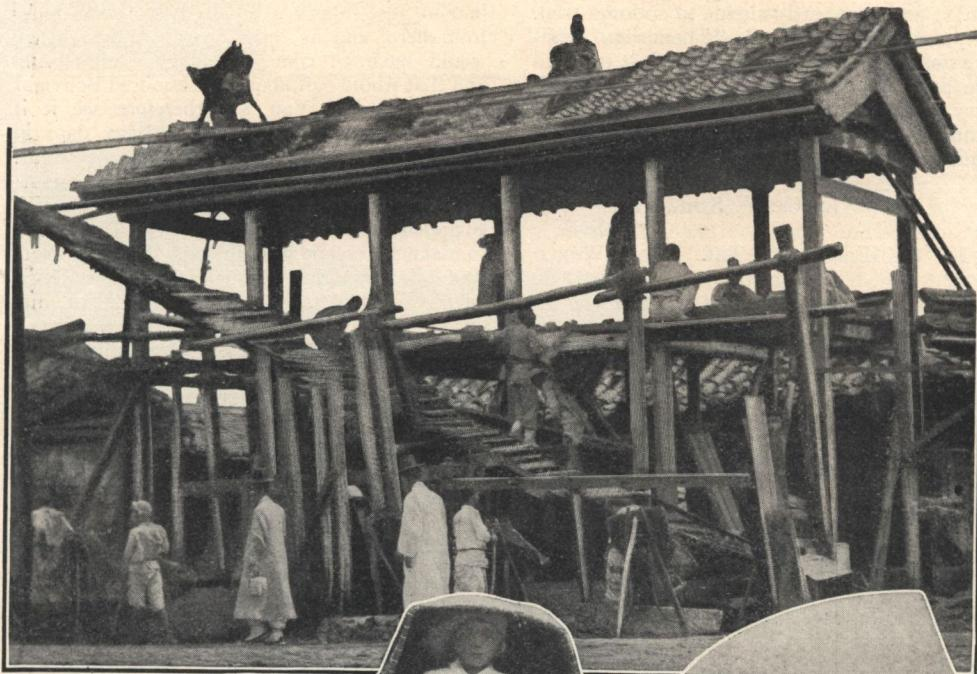
Korean methods of building—The roof is put on first of all, and the upper storeys are reached by a sloping gangway.
