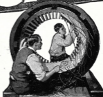
Student Winding Stator at COYNE
