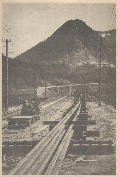
Long approach for easy loading. To transfer rail section from assembly line in the distance to flatcar in foreground, GN engineers laid down a ramp of graded rollers and placed their train on 2.2 percent slope. Steam winch and steel cable provide power
