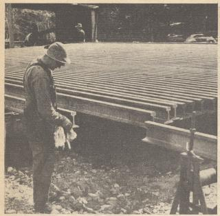
Continuous rail for Cascade Tunnel—1326-foot lengths to replace the 39-foot sections laid down in 1929—cost the Great Northern approximately §189,000 plus two months of intensive welding and polishing on a slope near Scenic, Wash. The figures on material and work expenditure, however, do not tell the whole story. Photographically recorded here are the complex operations preceding the driving of the "last spike" in midJuly in the four miles of continuous rail starting at the bore's east portal
