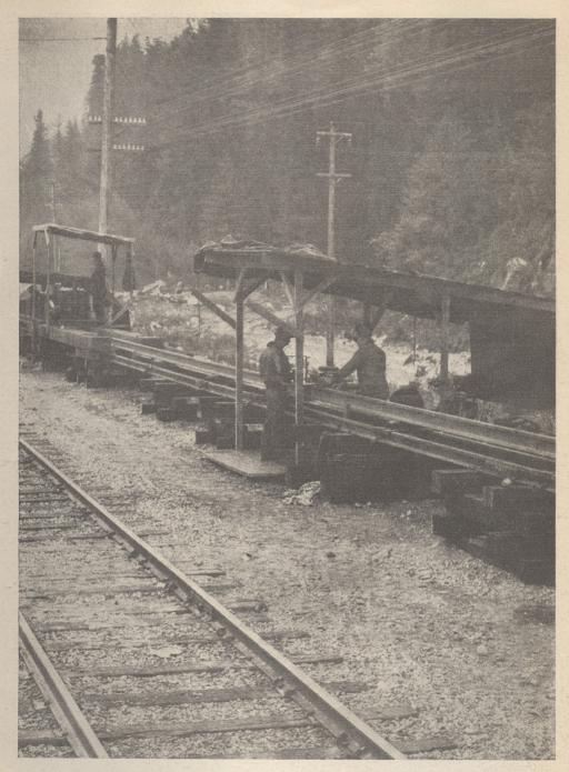
tunnel conditions give abnormal wear. Since 1929 only five of the more than 17,000 placed between portals have been removed, these being located over a soft spot where there was a wet condition and
