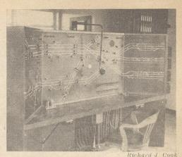
Operator at the new interlocking plant at Fostoria (Nickel Plate) station never has to leave his chair to line up the routes. Board is of the latest push button type
