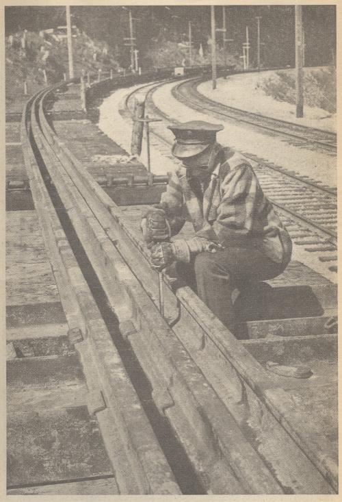
Clamping down on a 75-ton load. Before the special train gets under way, a worker tightens the bolts of a clamping device which secures each of the rails at a point midway in its length and prevents lateral motion later on. Three is the maximum load for Cascade Tunnel, though individual rollers for 12 rails have been installed
