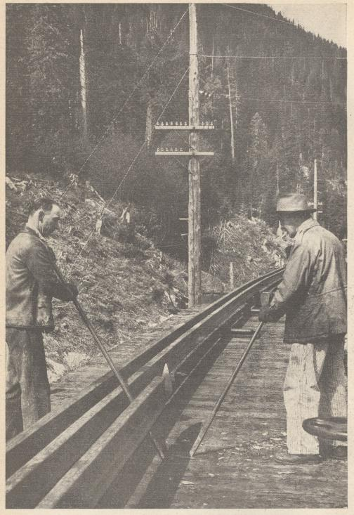
Margin for error is slight, as the 1326-foot steel bar inches its way forward along the cut of 25 roller-equipped cars under the watchful eyes of two railroaders. A shoe fixed to the lead end makes progress over portable rollers easy; the steam winch is still doing the heavy work. As soon as the rail is in place, a second coating of preservative will be sprayed on
