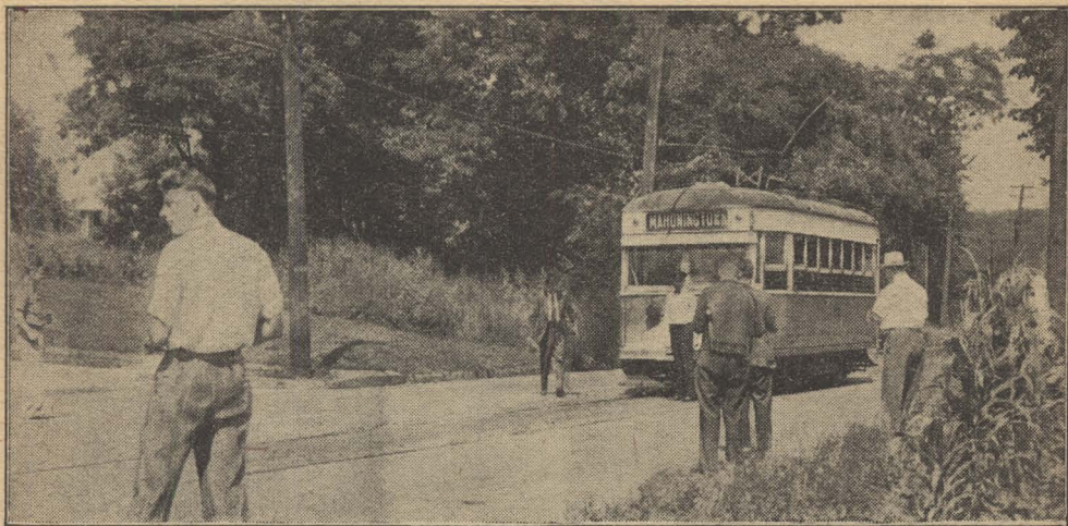
Photo by C. W. Burns, 403 15th St., N. W., Canton, Ohio
