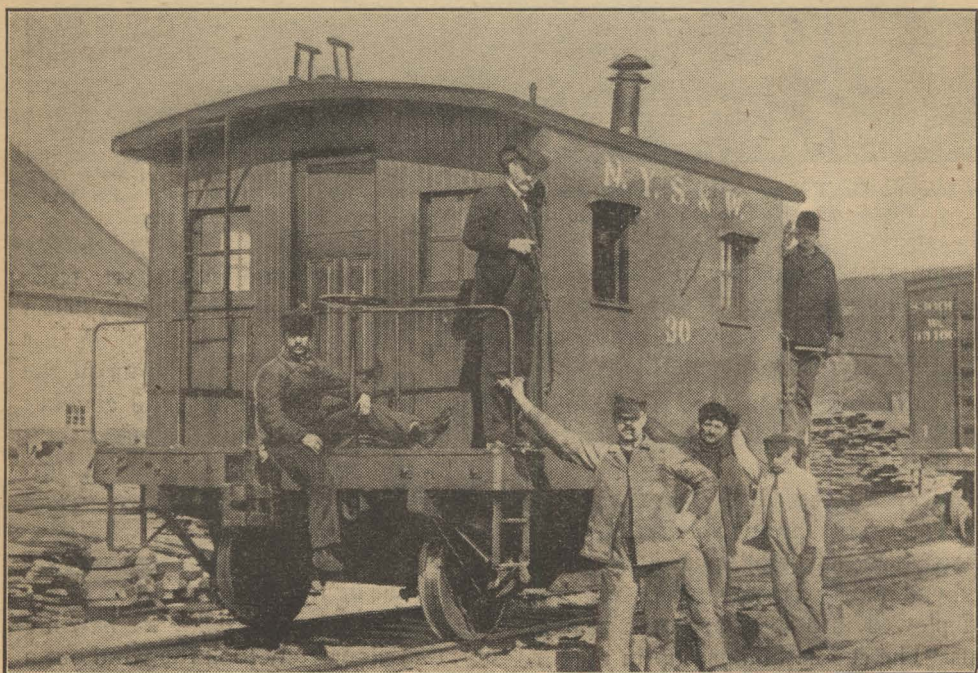
The Above View of a Crummy on the New York, Susquehanna & Western also Was Made on a Winter's Day; but When or Where, Nobody Seems to Know. It Was Loaned to Us by a Charter Member of the Railroadians of America in the Hope That Some Reader Might Identify at Least One of the Six Men Pictured Here
