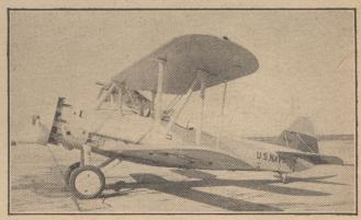
This new Vought O3U-3 powered with a 600-h.p. "Wasp" is the Navy's best bet where two-seater fighters are required. This is am improvement on the old Corsair and packs high speed and many high-caliber guns fitted under the cowling and inside the wings. Note the heavy gun in the upper center-section.
