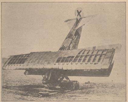
Photo by R. R. Martin Here's one to show you how the Fokker wings were made. This D-7 was shot down on the Western Front and, in tearing off the insignia, the captors disclosed the detail of the construction. Note the leading edge stiffening formers which were made of strips of three-ply.
