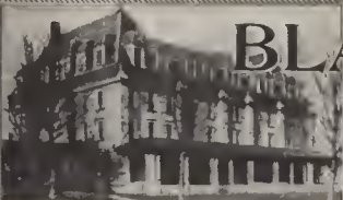
One of the 7 Buildings
