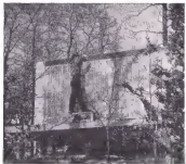
Front wall is hinged to roof beam, swings out, up to form porch roof.
