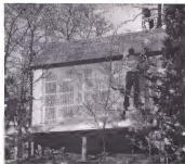
AFTER only one day's work, roof is up, provides overnight shelter.
