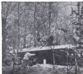
Floor sections are laid down and bolted to cedar-post foundations.
