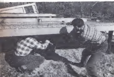
To insure level floor, wedges are inserted under panels where needed.
