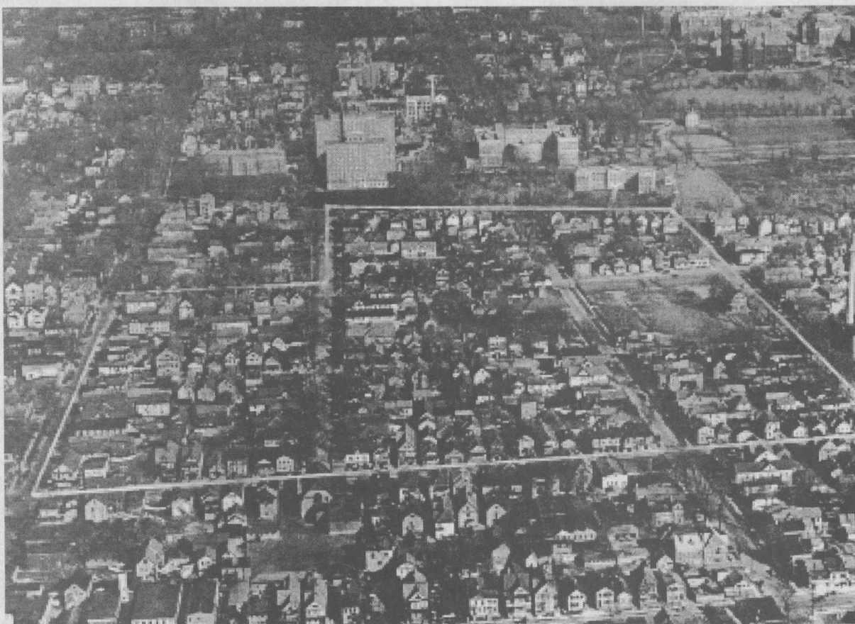
Air view of site of Syracuse Housing Project before demolition
