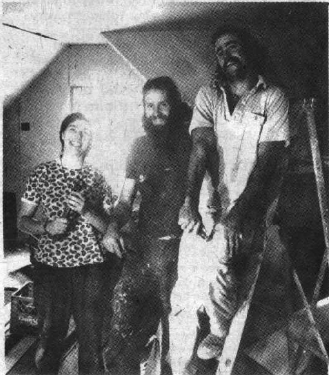
House remodeling crew - Susie Gaines, Dave Coons, Joe Horsington - upstairs.
