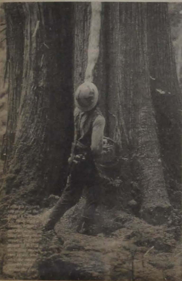
LOGGER FELLING MASSIVE CEDAR
