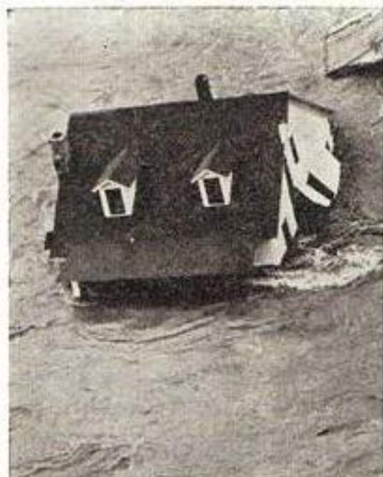
No palaces were washed away, but the home into which many a worker had built his hopes, went drifting with the flood.
