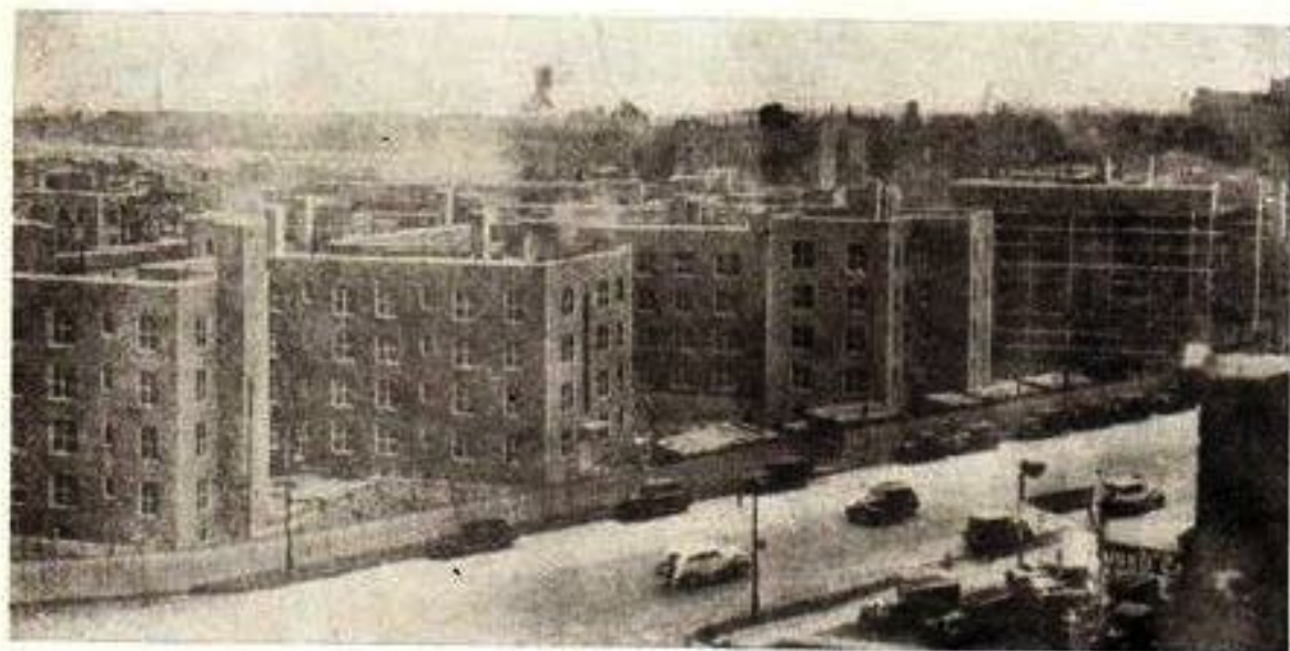
The PWA workers who put up these apartments at 153rd Street and the Harlem river, designed for low income groups to solve New York City's housing problem, will not live in them—for prospective tenants must show a bank account and have a job.
